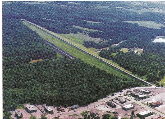
Aerial photograph taken in 1993 shows Englewood Dam as it appears today under U.S. Route 40. Source: Miami Conservancy District
