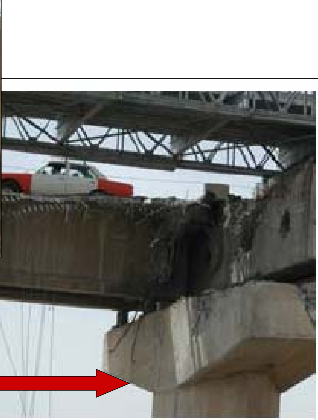
Damaged Pier 7, west end
