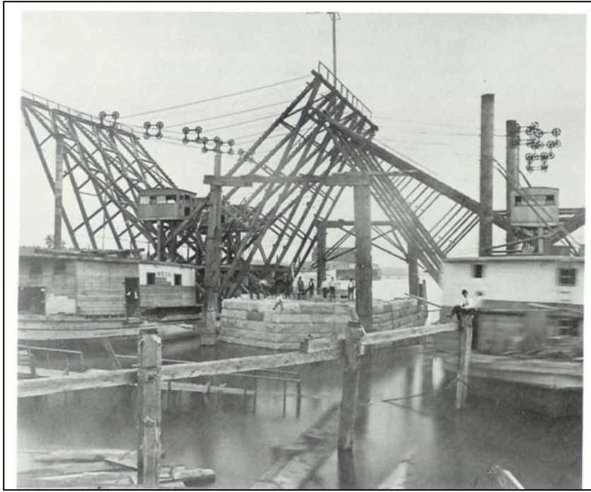
Derricks and Pontoons for the East Pier
