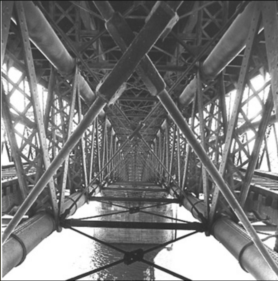
Assembled Ribs Showing Couplings and Braces
