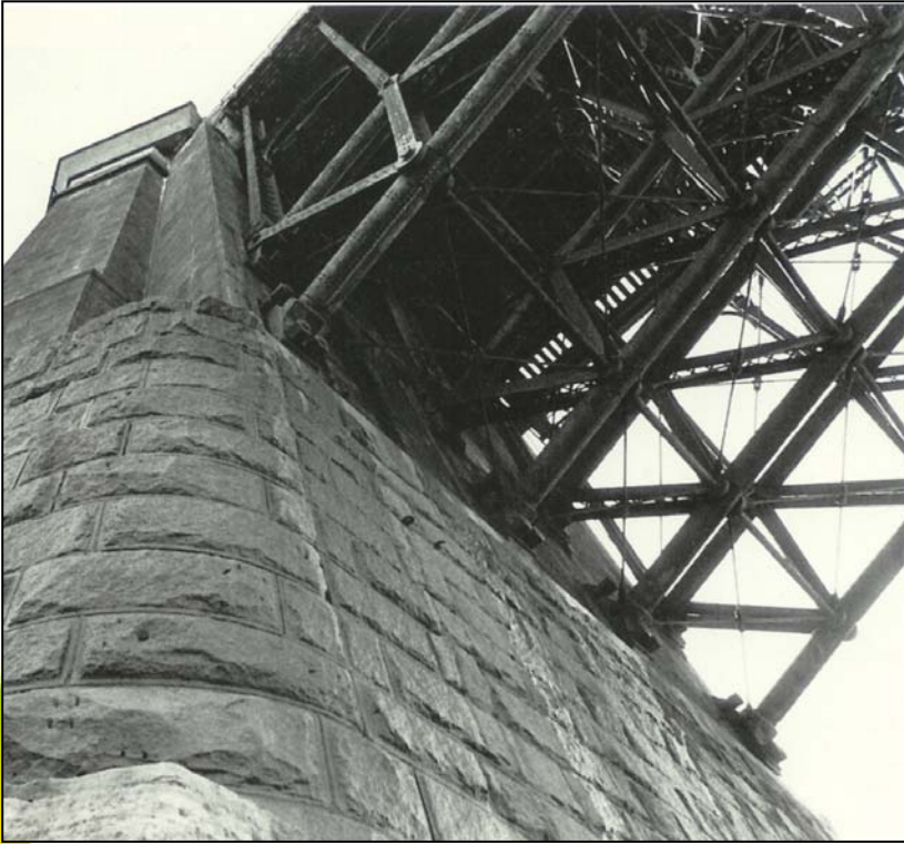
Superstructure Connection to Masonry
