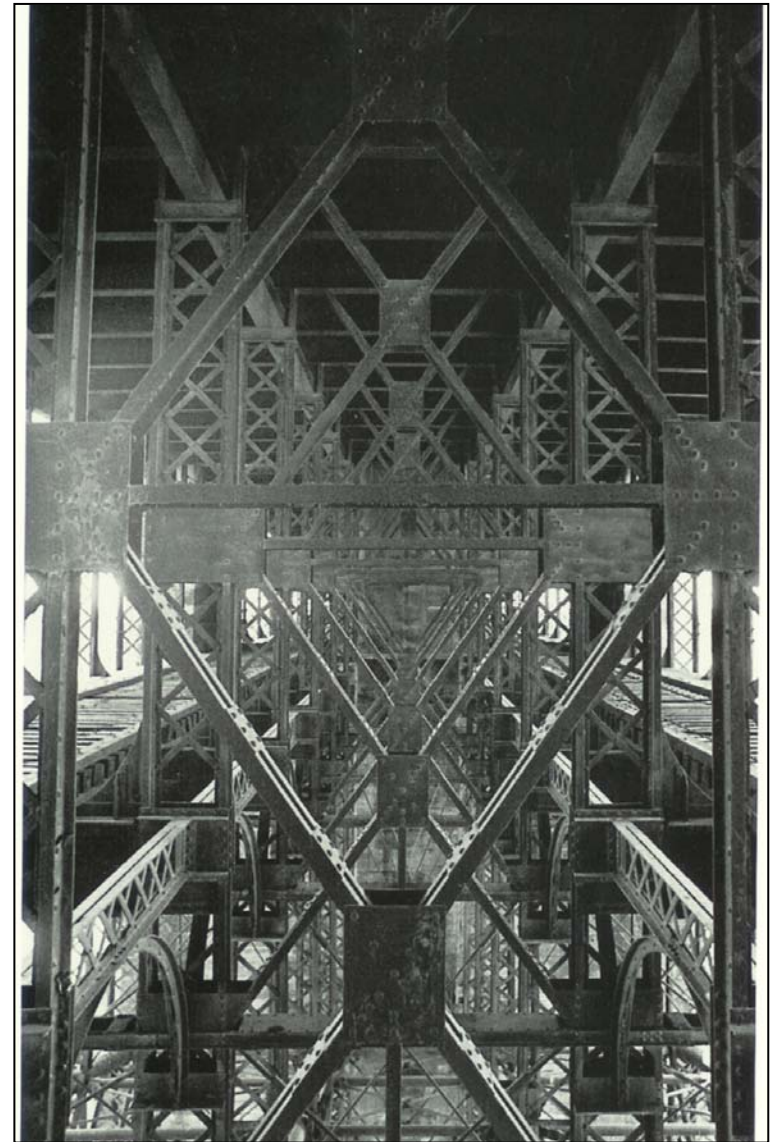
Road Deck Support
