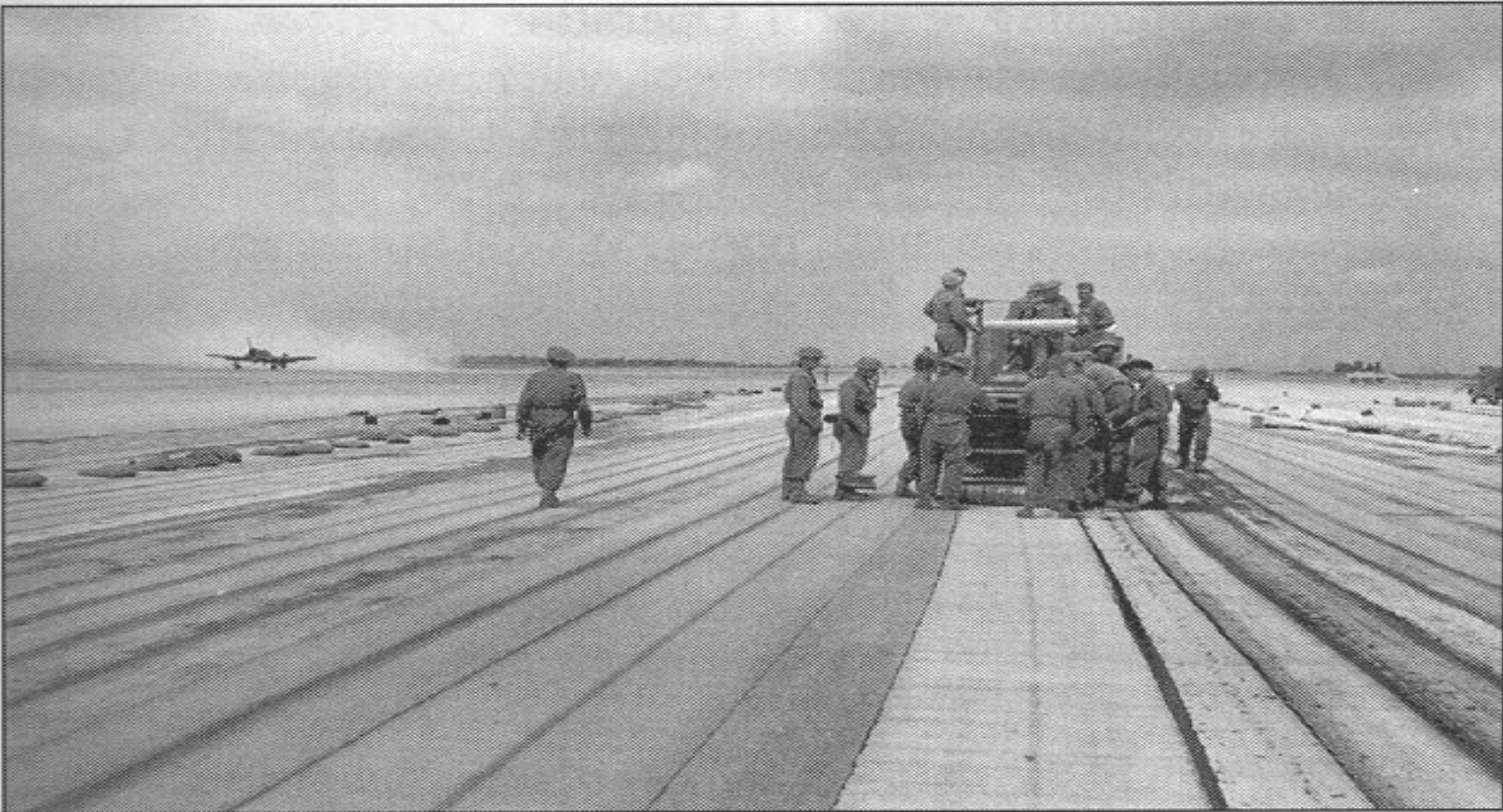
Figure 7. Landing strip in Normandy being constructed from Prefabricated Bitumenized Surfacing. Note the flat surface of the Calvados plateau, ideal for temporary airfield construction, and the dust being generated from dry loessic soil by a Typhoon taxiing across an “unpaved” area. (Copyright, The Imperial War Museum, London: photograph CL468.)
