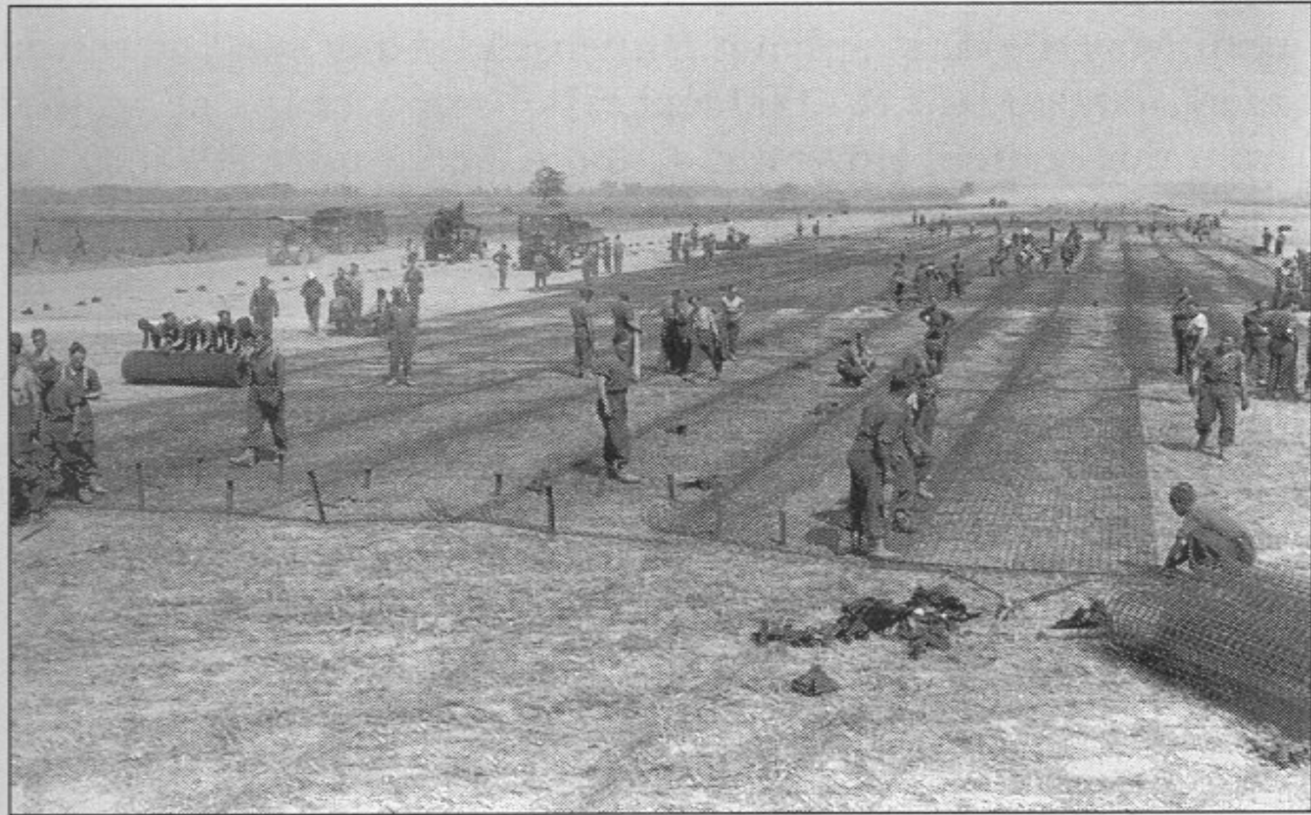
Figure 6. A British landing strip in Normandy being constructed with Square Mesh Track, on August 10, 1944. (Copyright, The Imperial War Museum, London: photograph CL710.)
