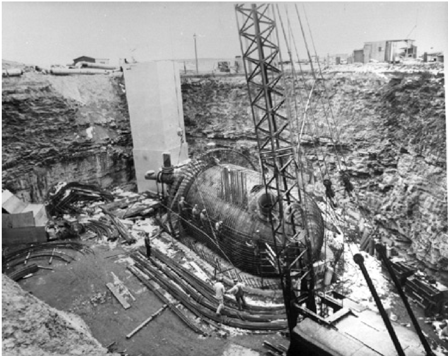
Launch Control Capsule module under construction at Malstrom AFB, MT in Nov. 1961
