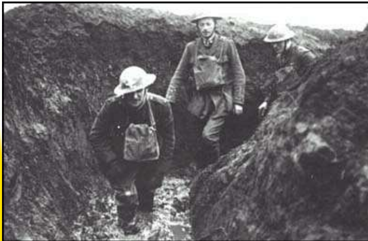
Officers walking through a flooded communication trench.
