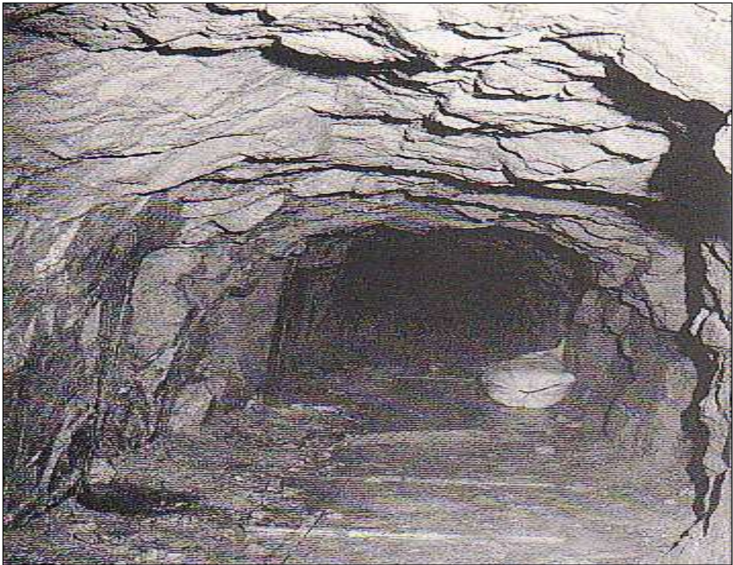
View inside Tunnel #4
