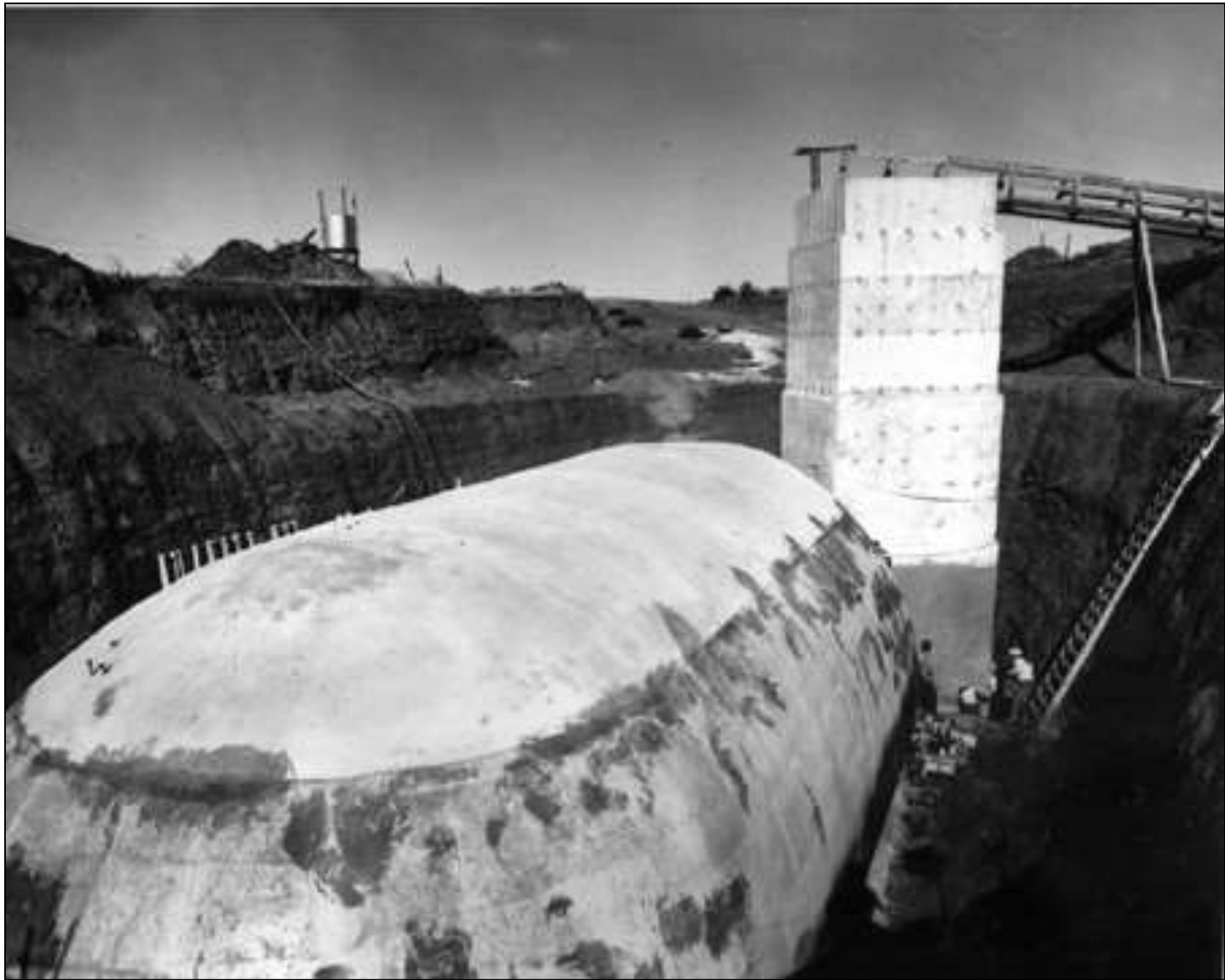
Close up of Launch Control Capsule under construction at Ellsworth AFB, SD in Sept.1962
