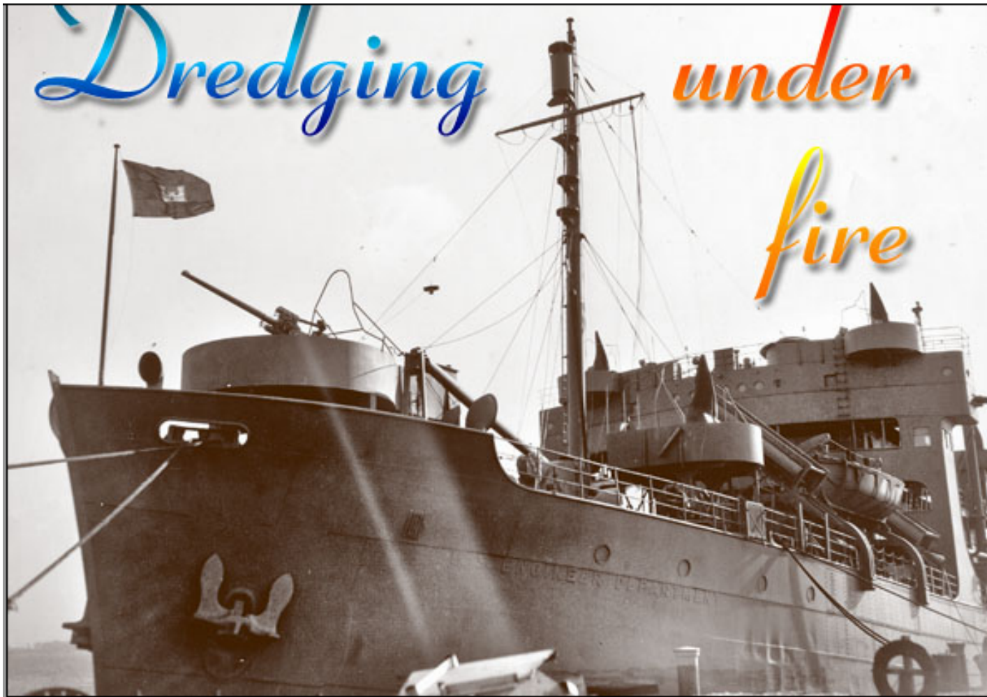
Port Restoration - WWII
