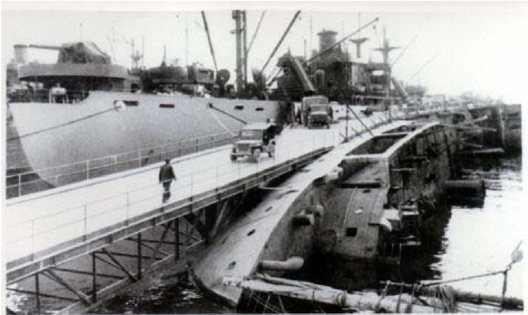
SUNKEN SHIPS in the harbor at Naples converted into piers for the berthing of Allied ships.
