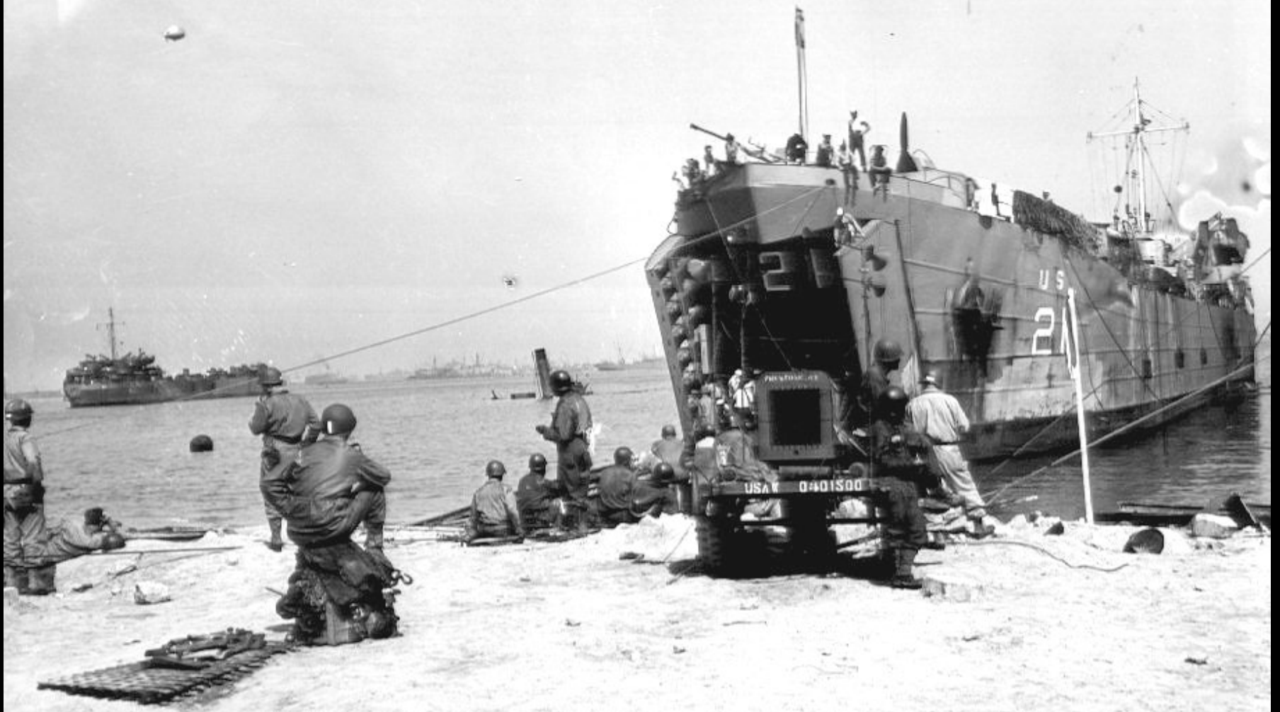
Positioning LST on temporary quay for unloading rail cars
