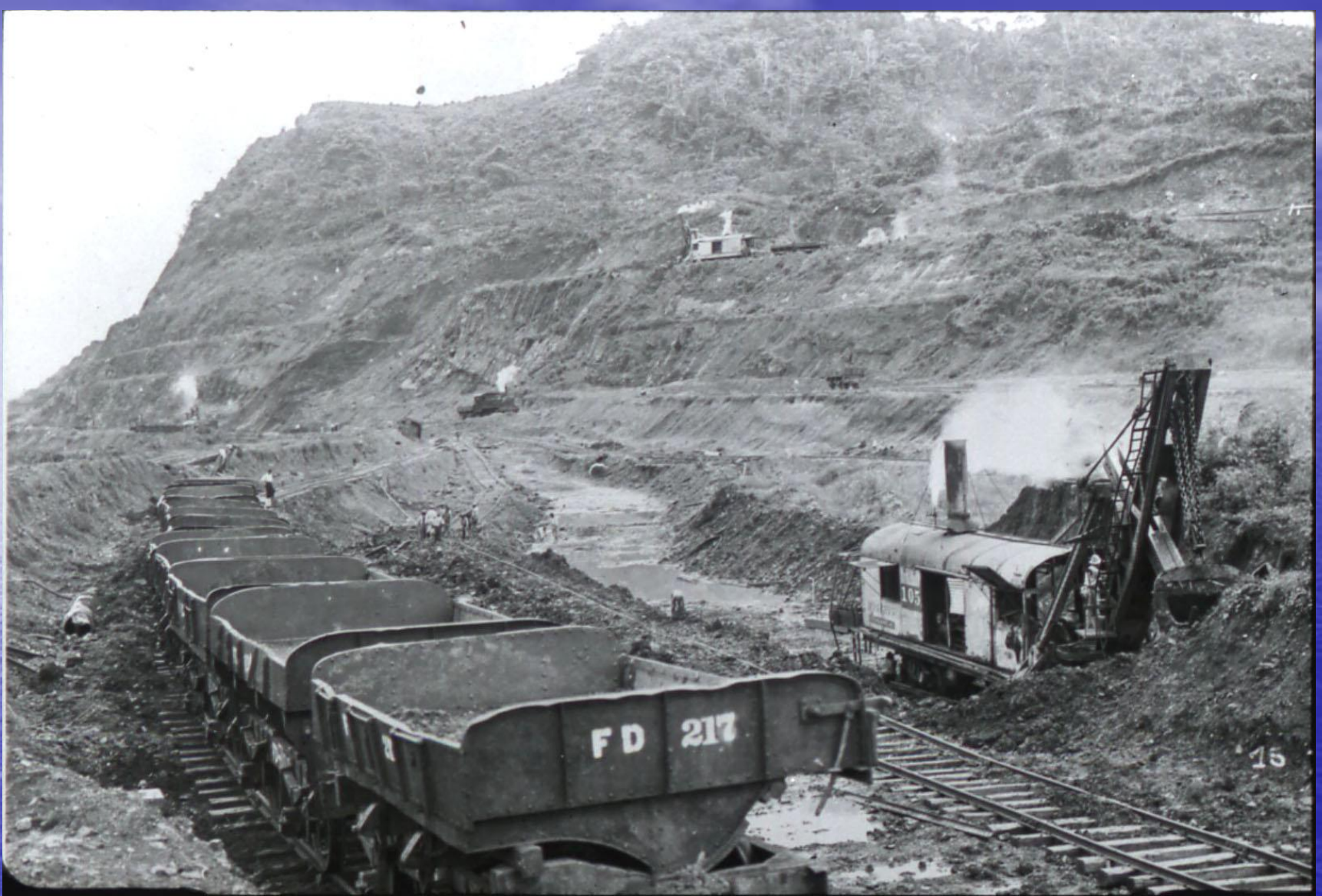
● Close-up view of the rail-mounted shovels excavating slide debris at Culebra. Side-dumping gondola cars in foreground.
