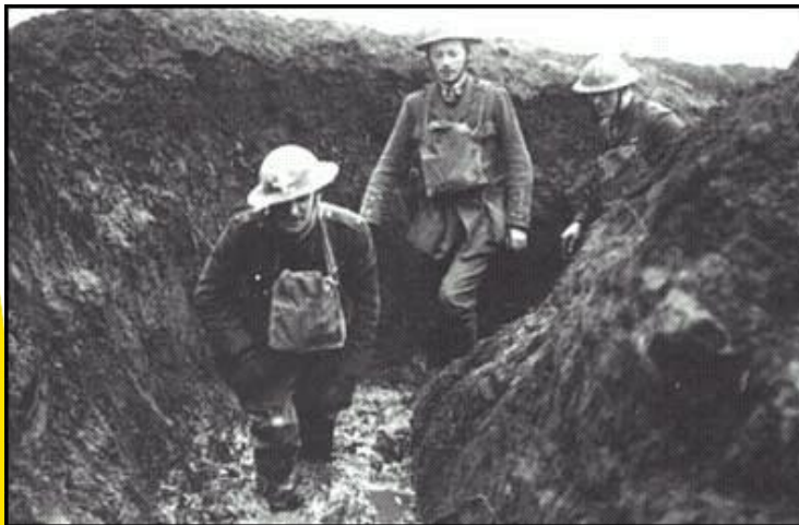
Officers walking through a flooded communication trench.
