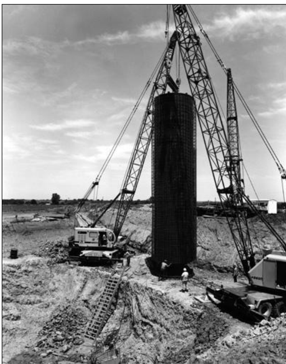
Construction of Minuteman Launch Silo B-11 at Whiteman AFB, MO on June 18, 1962
