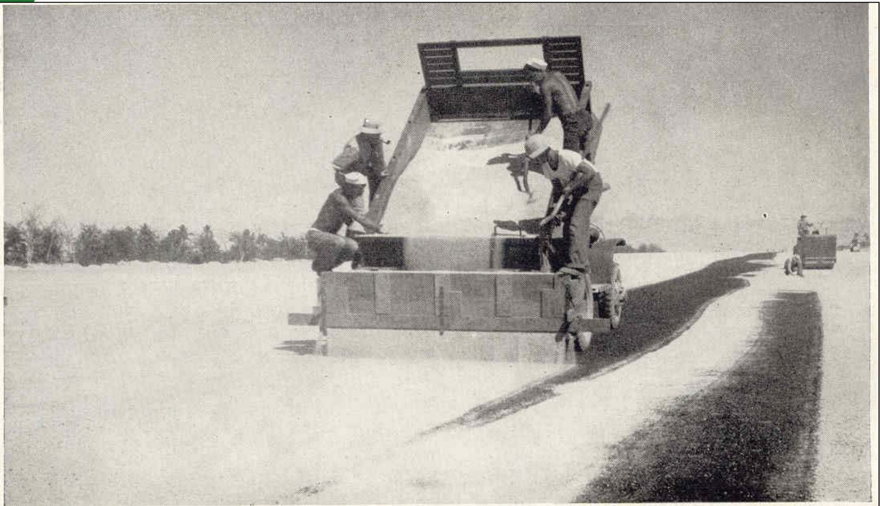
5. Surfacing with finely crushed coral – twelfth day.
