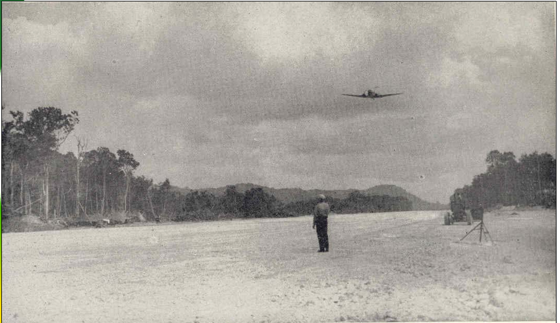
6. Bringing in the first plane—fourteenth day. On many fields the coral provides a sufficiently hard runway; other fields require the Marston mat. (Official U. S. Navy Photo)
