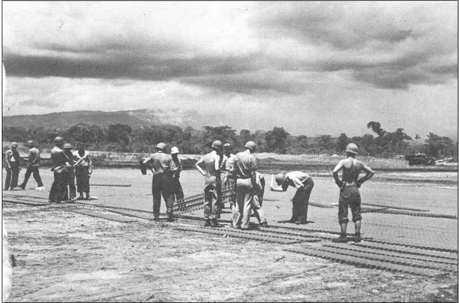
Repairing Marston Mats (PSP) at Henderson Field on Guadalcanal
