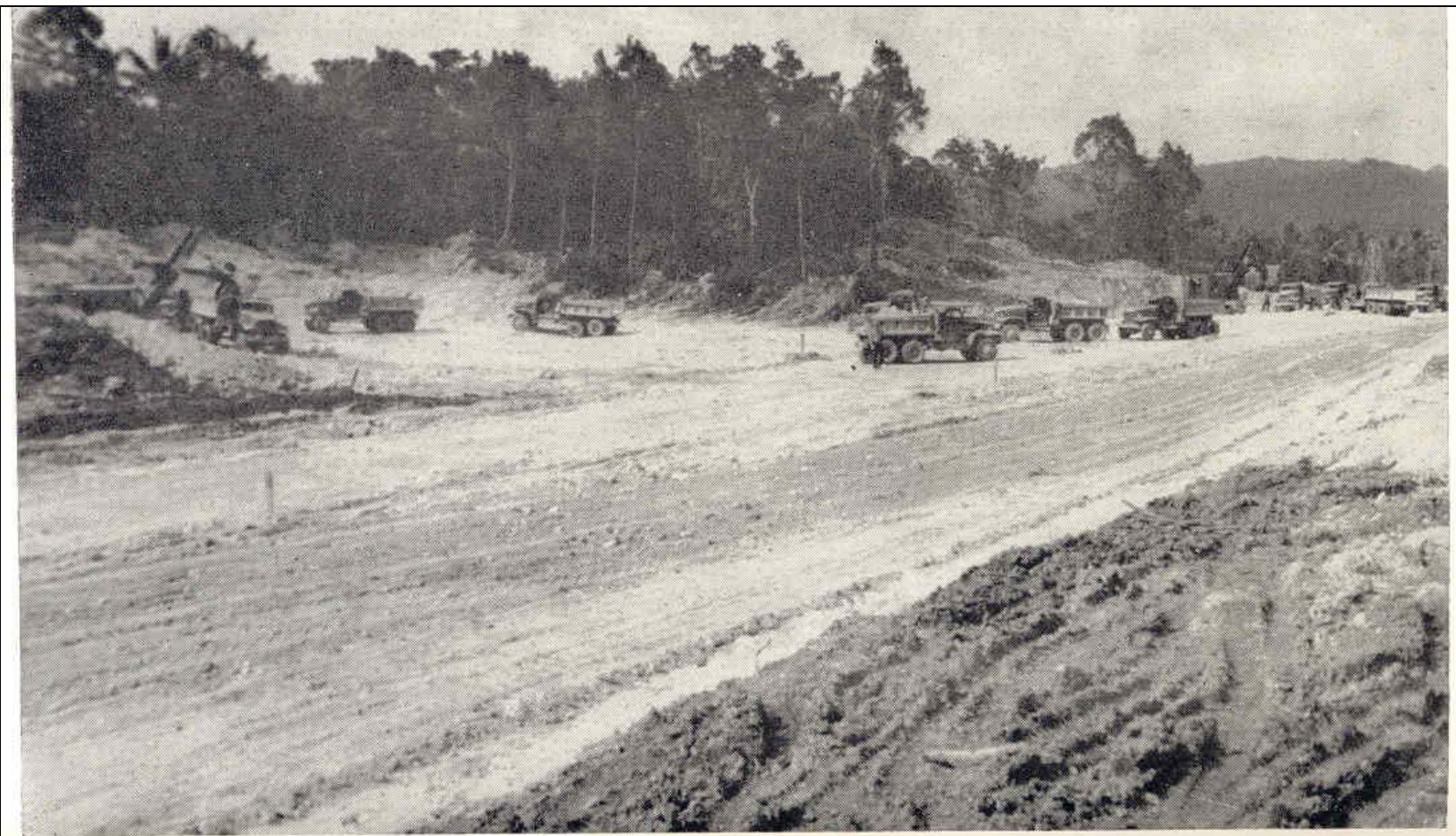
3. Excavating hardstands – parking areas – sixth day.
