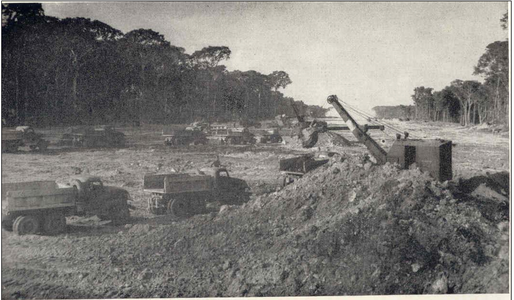
2. Removing the windows of earth piled up by the bulldozers — fourth day. (Official U. S. Navy Photo)
