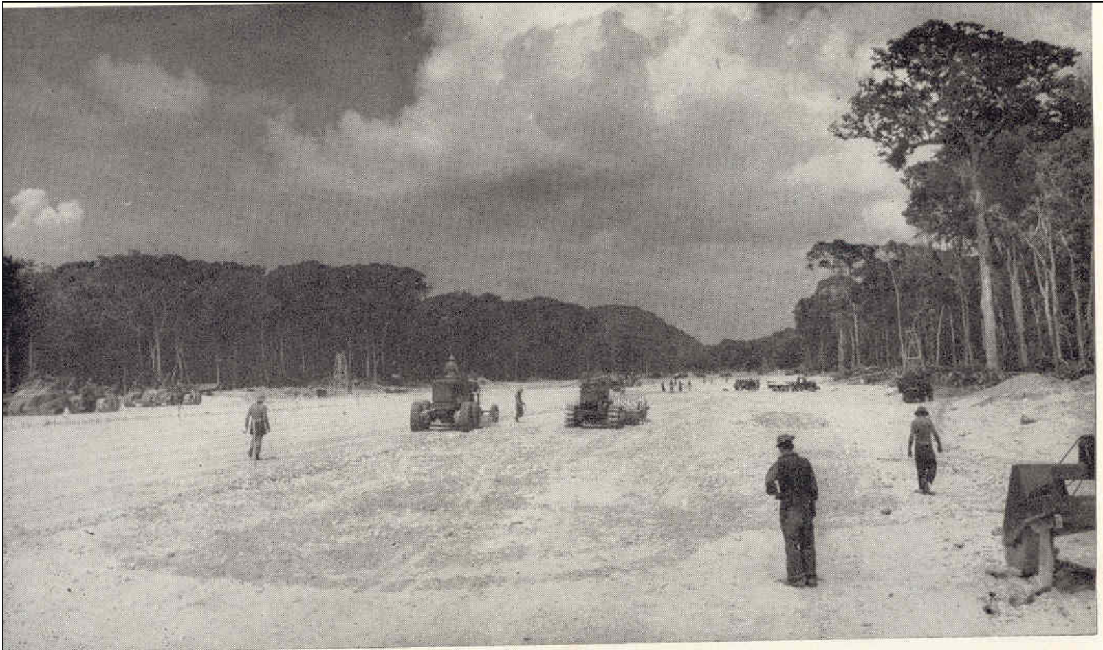
4. Grading and rolling with the "sheeps's foot" roller – eighth day. (Official U. S. Navy Photo)
