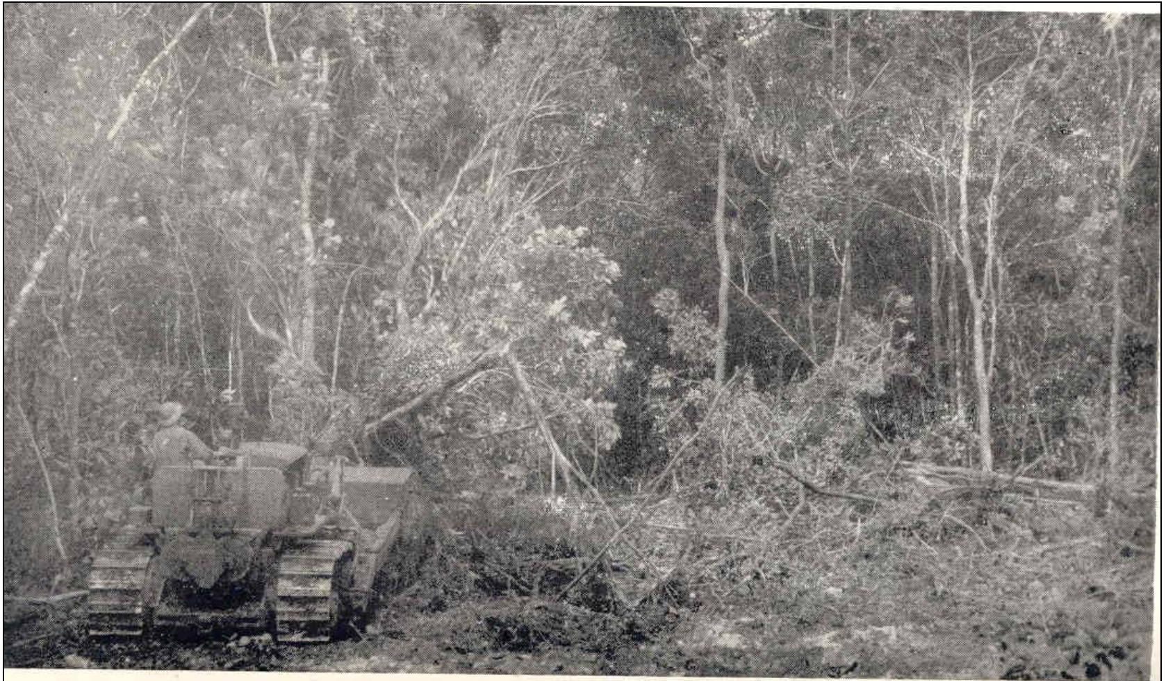
Here are six views showing the evolution of a jungle airfield. 1. Clearing operations – first day. (Official U. S. Navy Photo)
