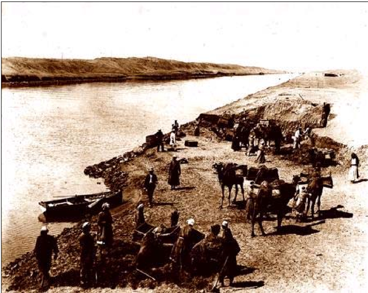
Excavation on dry land to widen the canal
