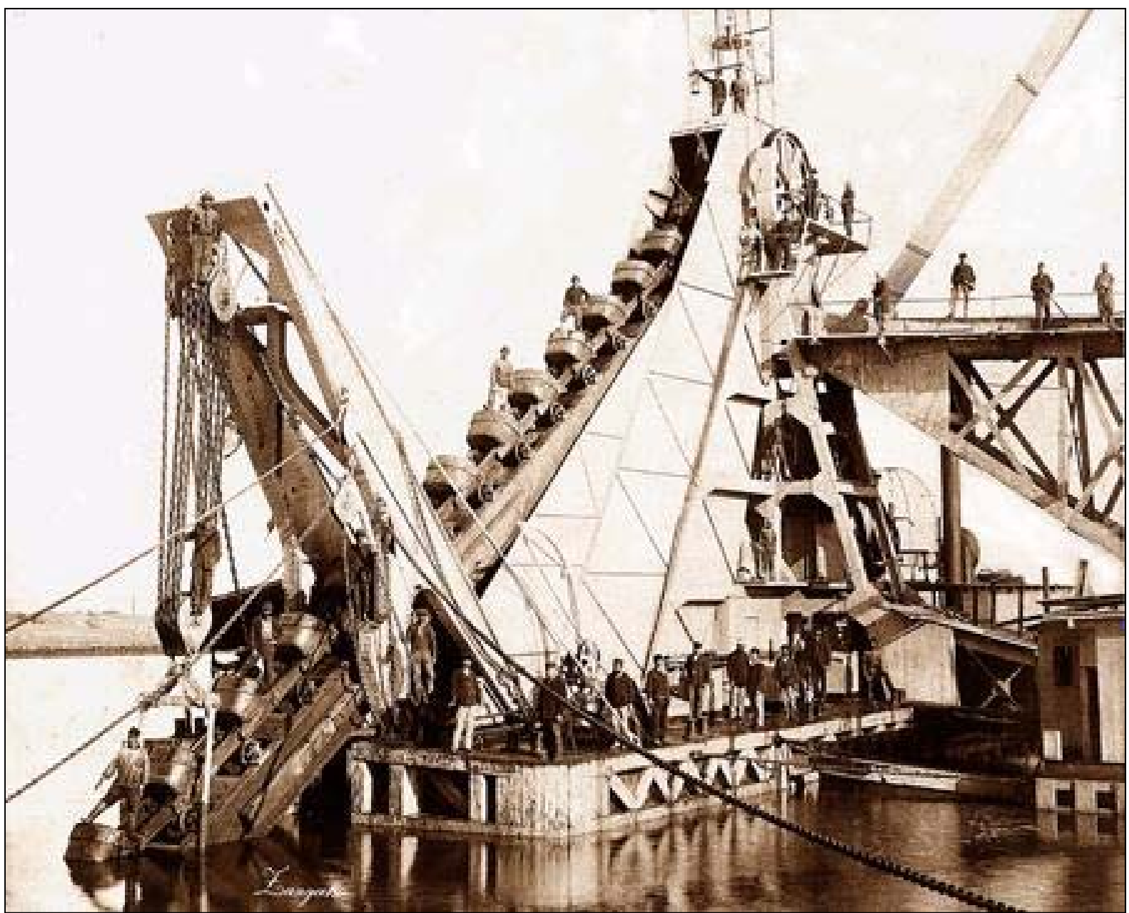
Close Up of dredger and crew.
