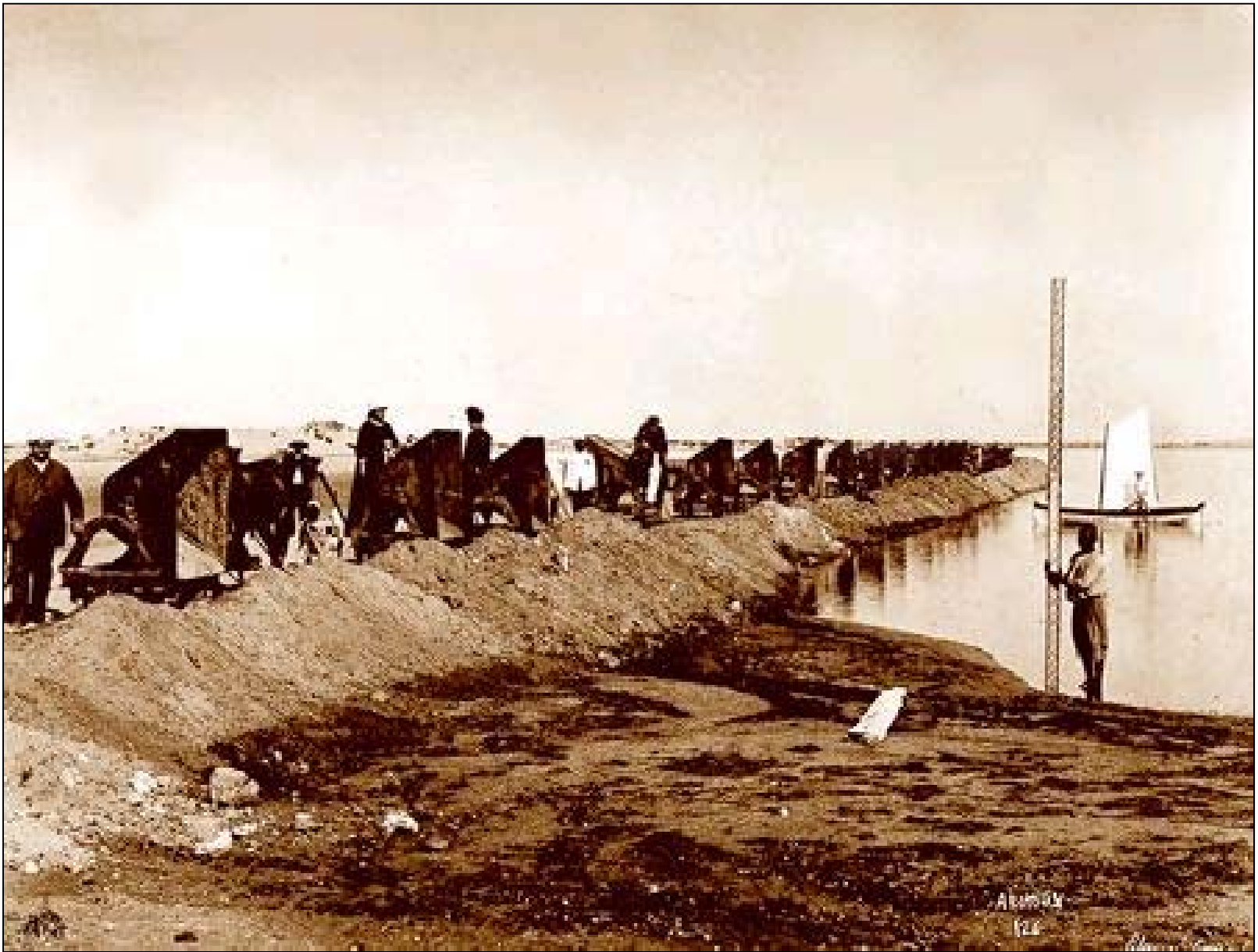
Work to widen the canal.
