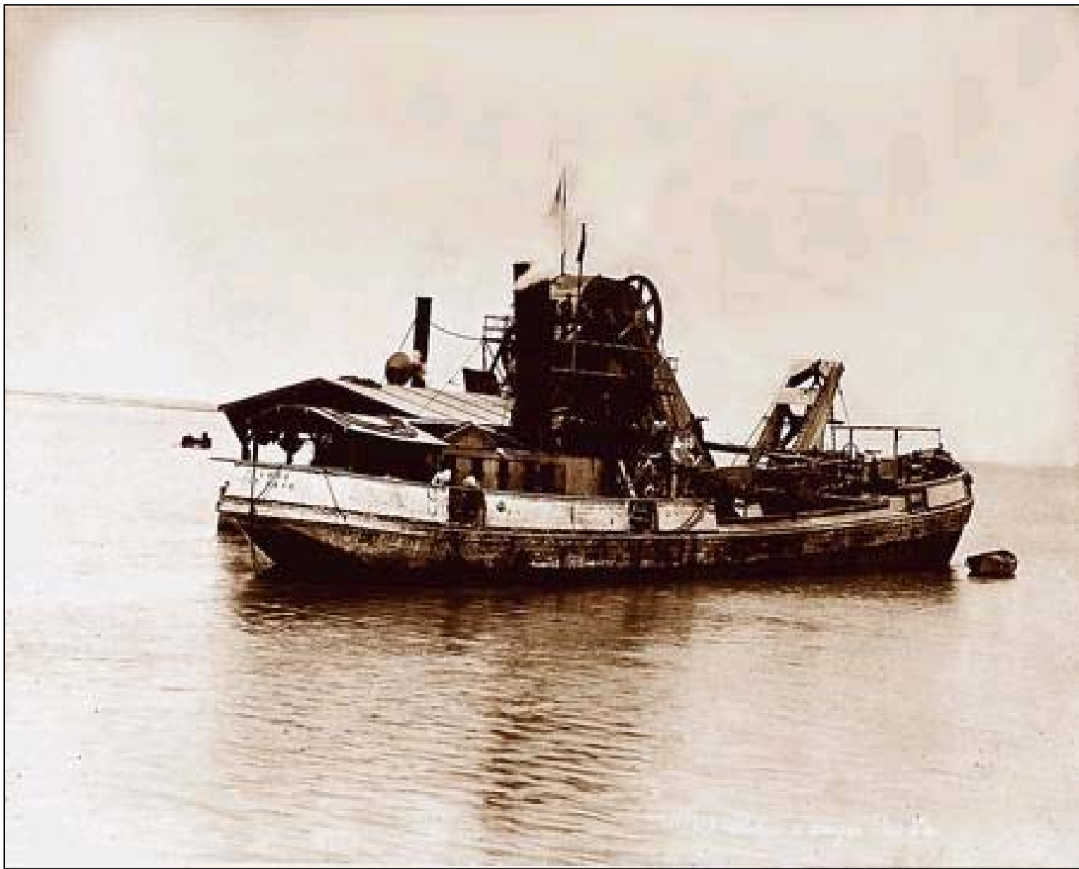
Dredger and Mud Barge.
