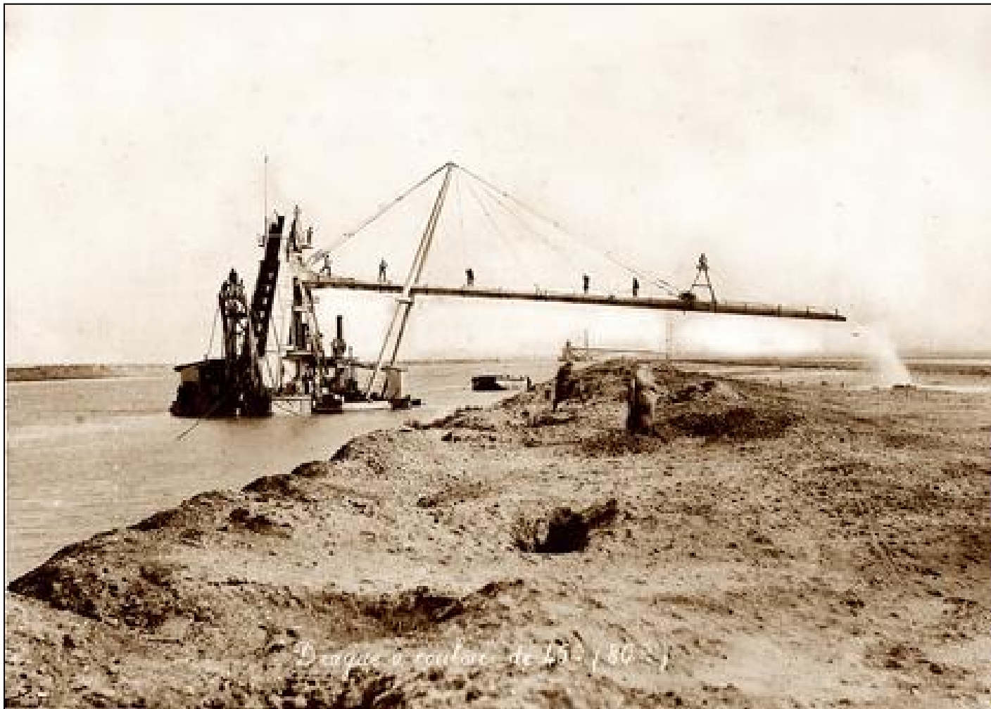
Dredger with a 45 meter chute.
