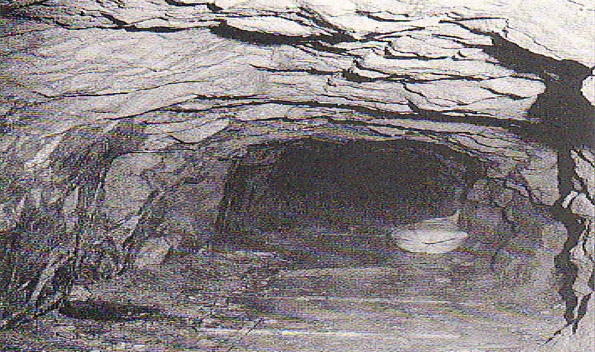
View inside Tunnel #4
