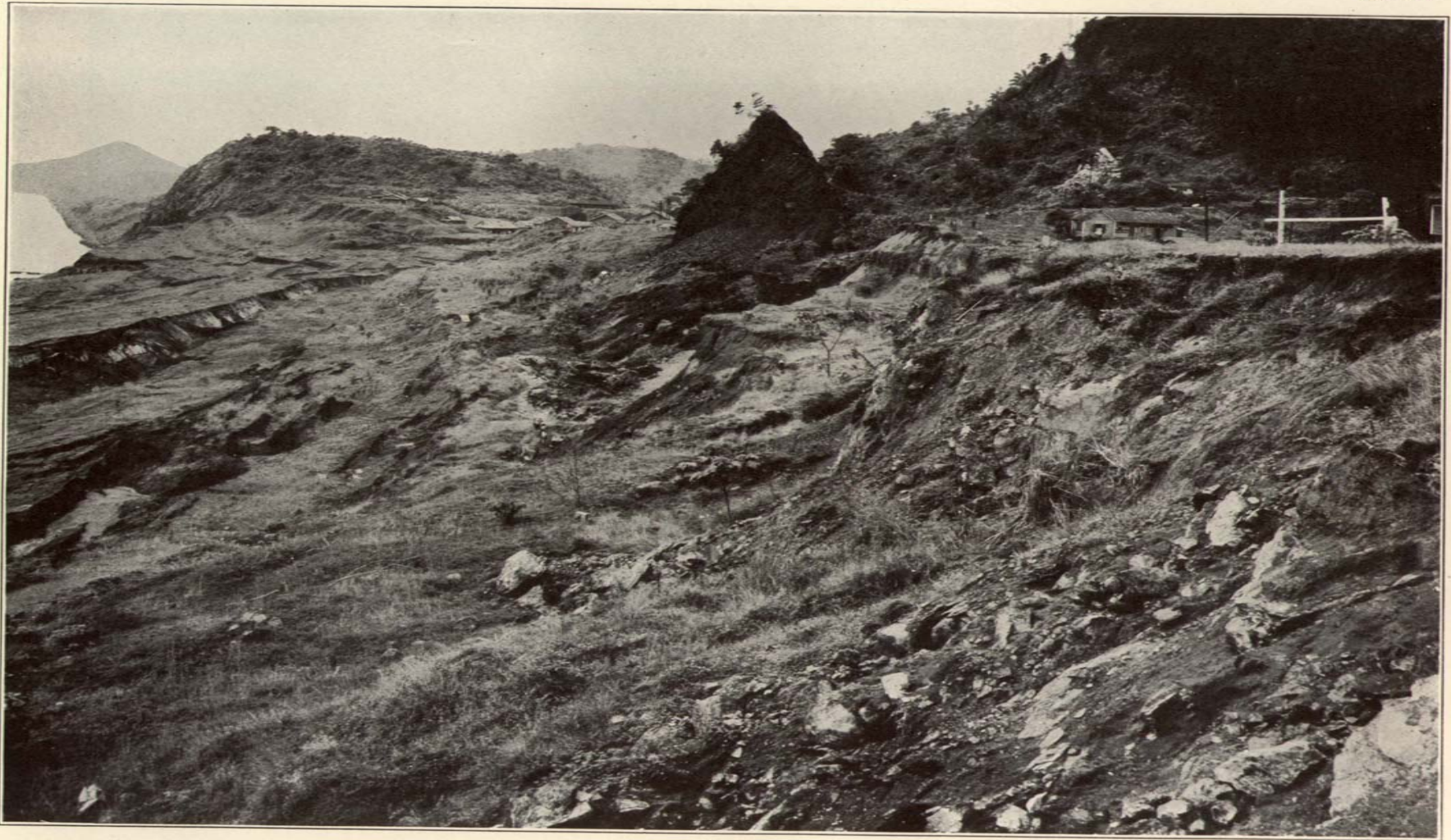
West Culebra Slide. View looking south from the edge of the slide, August 8, 1915.
