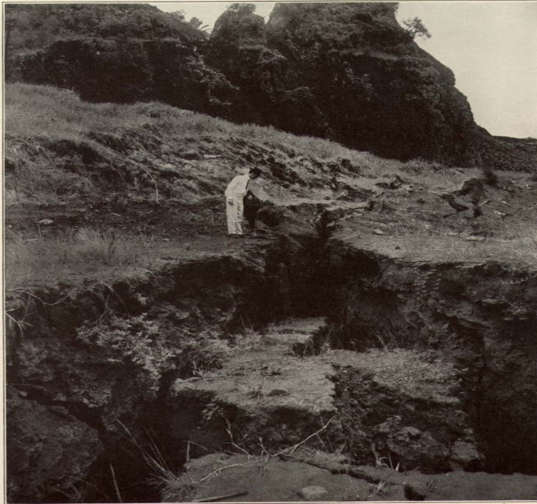
A fissure formed in connection with the breaking down of the face of Zion Hill, West Culebra slide area, August 8, 1915.
