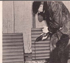
APPLYING MASTIC TO VERTICAL LAP
