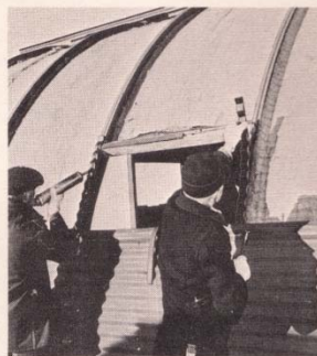
APPLY RUBBER OR ASPHALT STRIPS AROUND WINDOW FRAME
