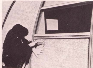
NAILING TO WINDOW SILL
