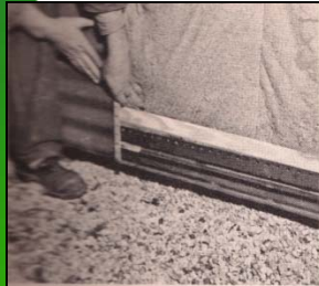
FIRST SHEET APPLIED 1 1/2" BELOW TOP OF JOIST
