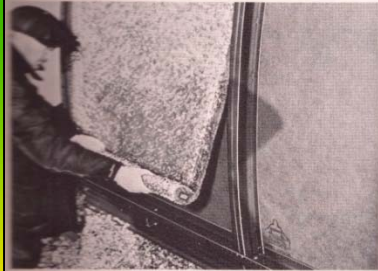
FASTENING INTO CHANNEL
