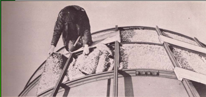
INSULATION APPLIED OVER MASONITE
