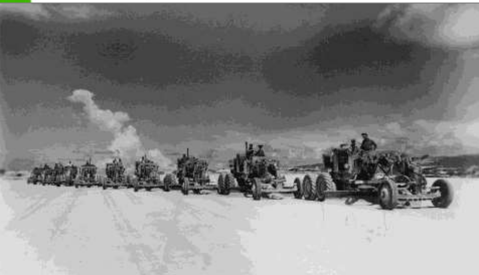
Spreading crushed coral topping for B-29 runways
