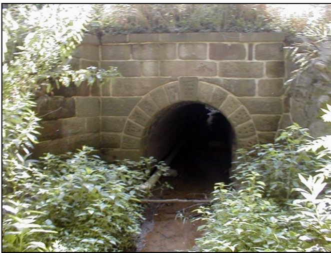
Above: Prior to the 1930s most culverts were constructed of masonry, like this one Below: Corrugated steel culverts were introduced in 1896. Segmented galvanized circular steel culverts (shown below) began to dominate practice in the 1930s
