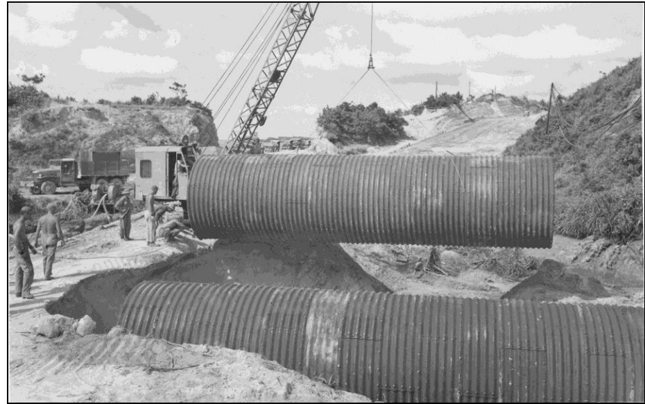
Little or no attempt was made in the early days to mechanically compact beneath the lower hemisphere of the circular culverts
