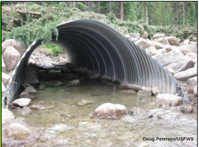
Correctly installed open-bottom arch culvert with footings
