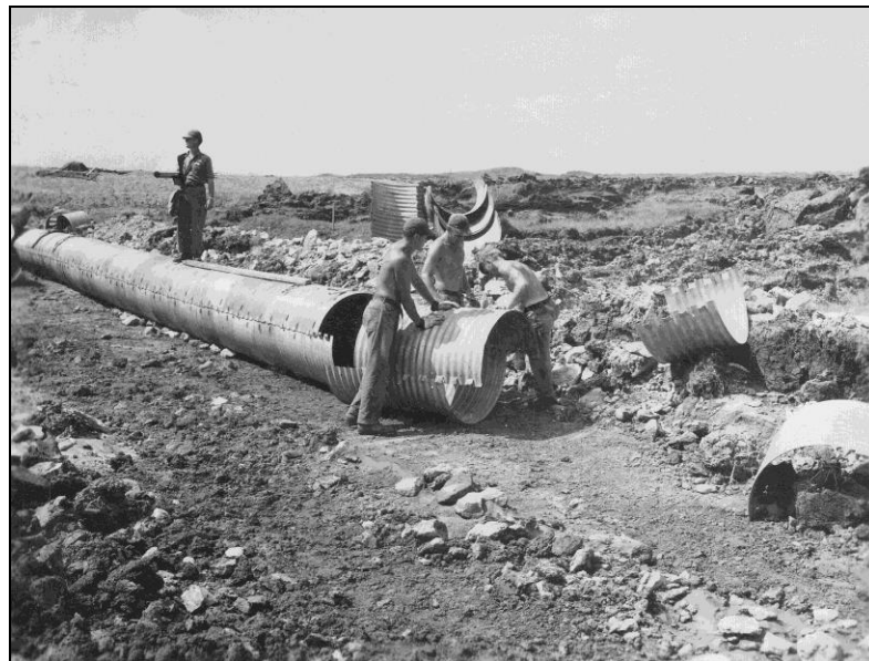
Above: Prior to the 1930s most culverts were constructed of masonry, like this one Below: Corrugated steel culverts were introduced in 1896. Segmented galvanized circular steel culverts (shown below) began to dominate practice in the 1930s
