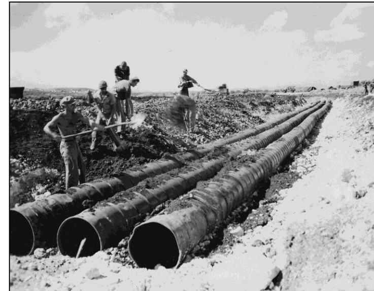
Little or no attempt was made in the early days to mechanically compact beneath the lower hemisphere of the circular culverts
