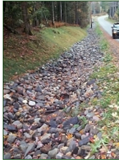
Neat-stacked rock-lined ditch
