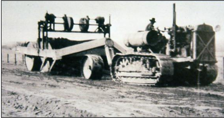
Old solid drum steel wheeled scrapper laying fill for the Bradley-San Ardo Highway in 1931
