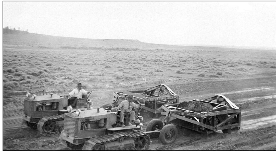
Old solid drum steel wheeled scrapper laying fill for the Bradley-San Ardo Highway in 1931
