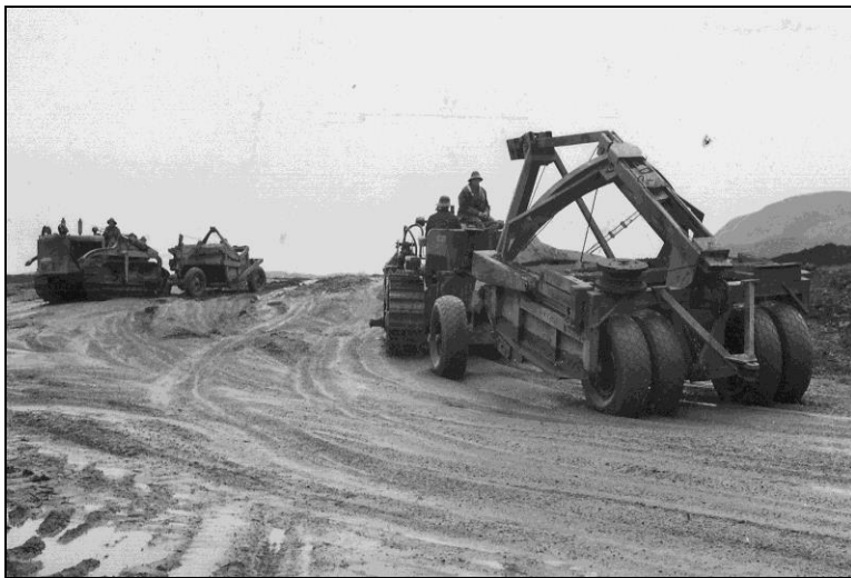
Old solid drum steel wheeled scrapper laying fill for the Bradley-San Ardo Highway in 1931
