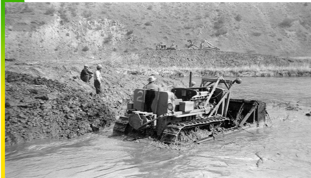
Caterpillar-LeTourneau dozer with power-takeoff cable control at a dam site in Montana in 1937.
