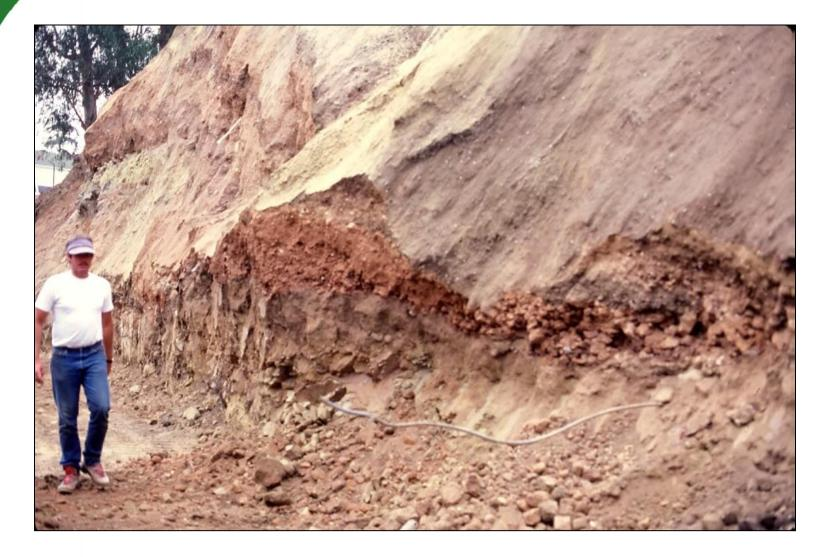
Keyways should extend through unconsolidated materials, such as older fill (shown here), topsoil, colluvium and the bedrock creep zone
