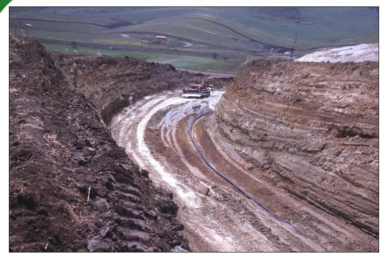
The toe-of-fill keyway is the most important part of an embankment. It bears the overall thrust of the slope and usually contains the lowest subdrainage.
