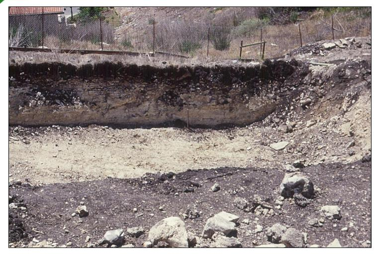
Modern grading ordinances required engineering geologic assessment of embankment keyways and deep foundation excavations to ensure that the assumed depths to suitable foundation material were adequate.
