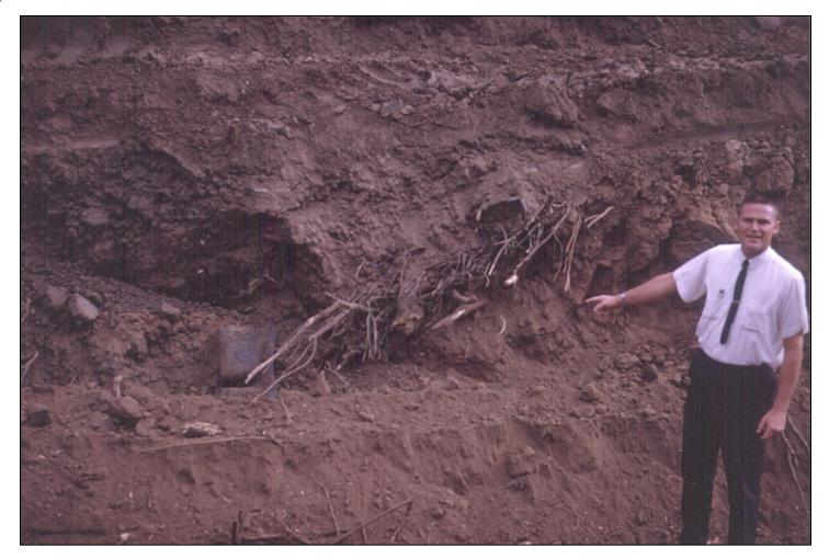
Another important aspect of grading inspection is to verify if deleterious materials, such as roots, trees and organic debris, are buried in the embankment. These can create unwanted zones of increased permeability and weakness.
