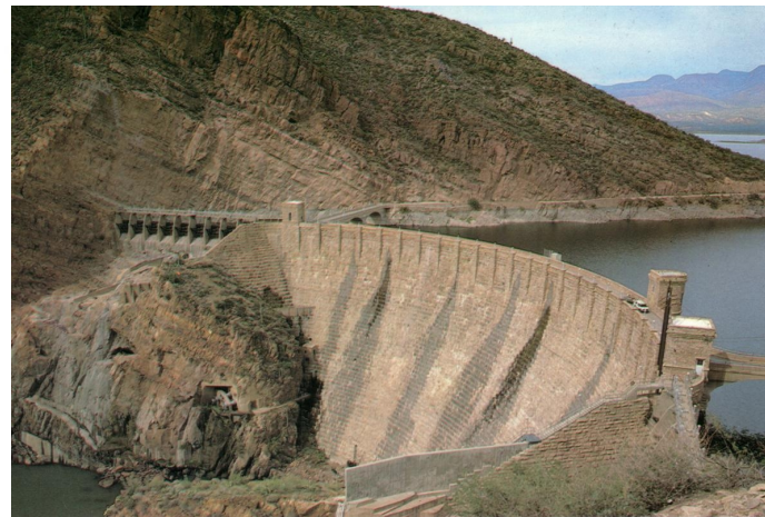
Roosevelt Dam on the Salt River in Arizona was constructed as a cyclopean masonry gravity dam by the US Reclamation Service in 1903-11
