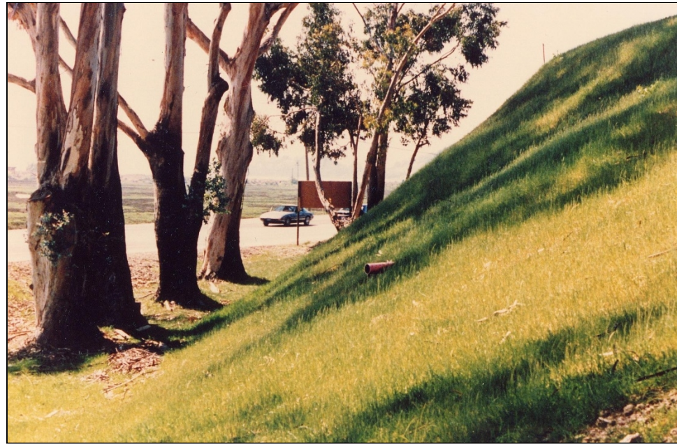
45 degree embankment slope along San Pedro Boulevard in San Rafael, CA
