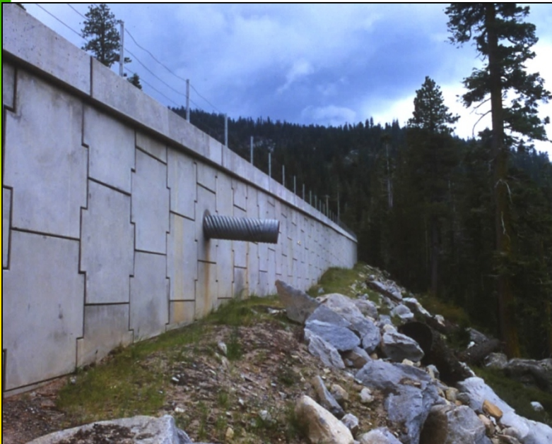
First Reinforced Earth wall in USA -1969
