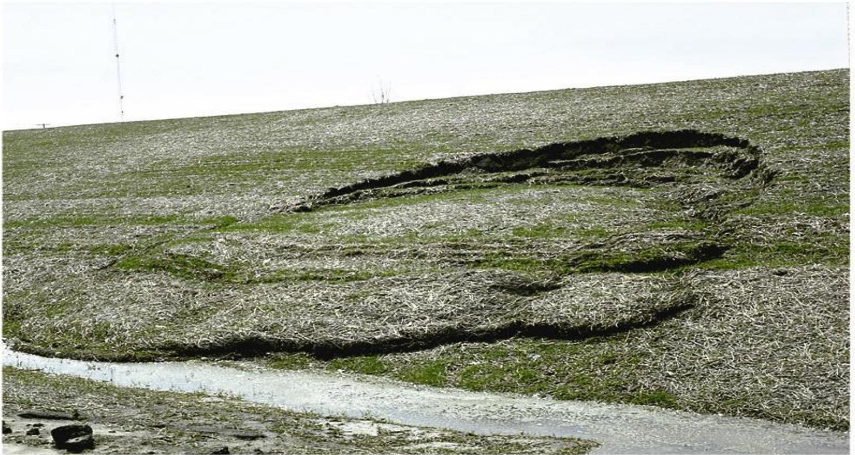
**Rotational slump-flow of a newly graded embankment along the westbound onramp of Interstate 44 in Rolla, MO. This slump was triggered by concentrated seepage along a single joint cluster, where they intersected a pervious bed**
