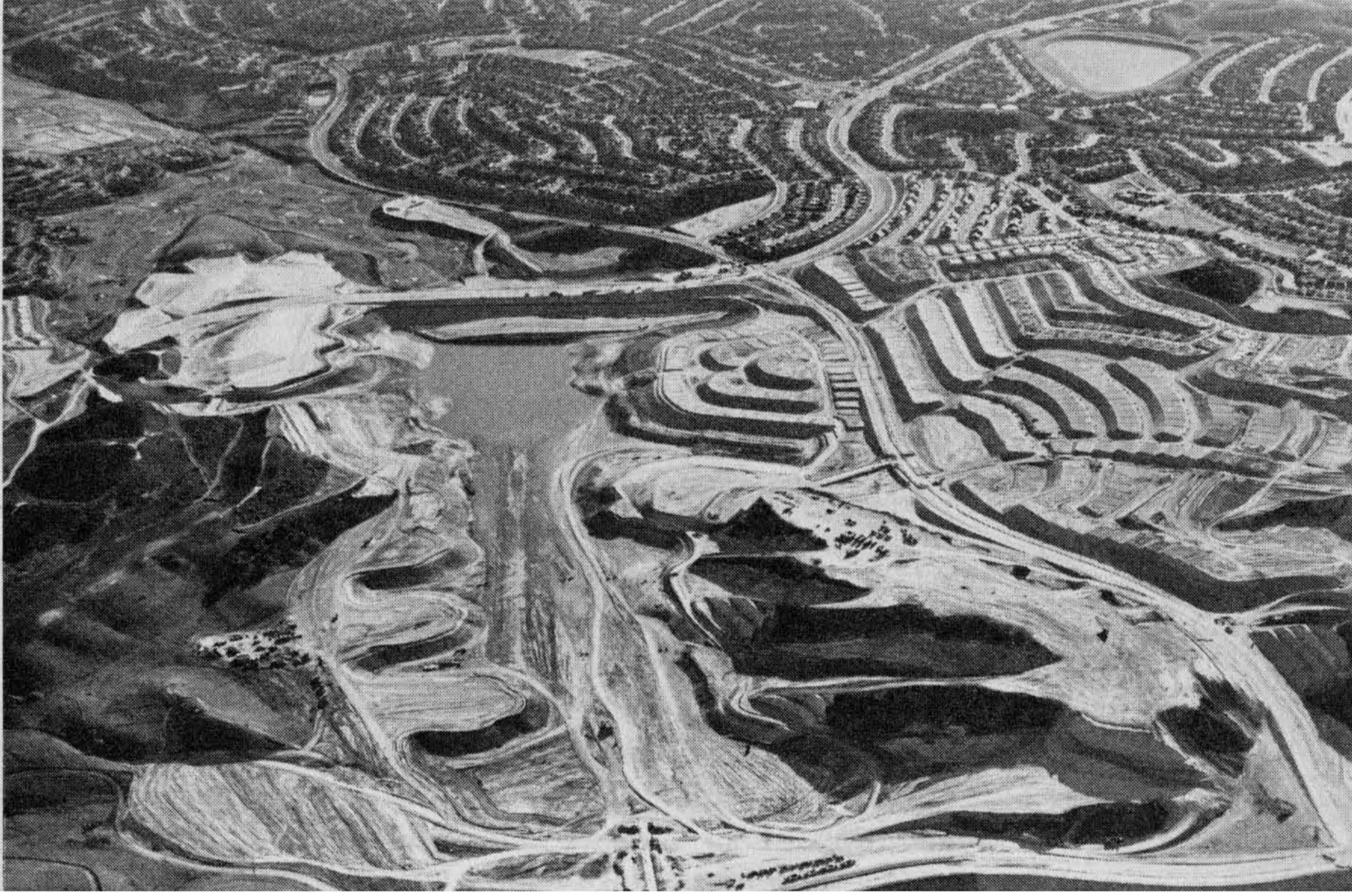
Figure 2.9 Lake Mission Viejo grading construction nearing completion, October 1976. Water is from rain runoff. The retention basin spillway is shown under construction in the center foreground. Rough graded residential sites are shown at right center. Photograph by Aerial Eye, Inc., courtesy of the Mission Viejo Company.
