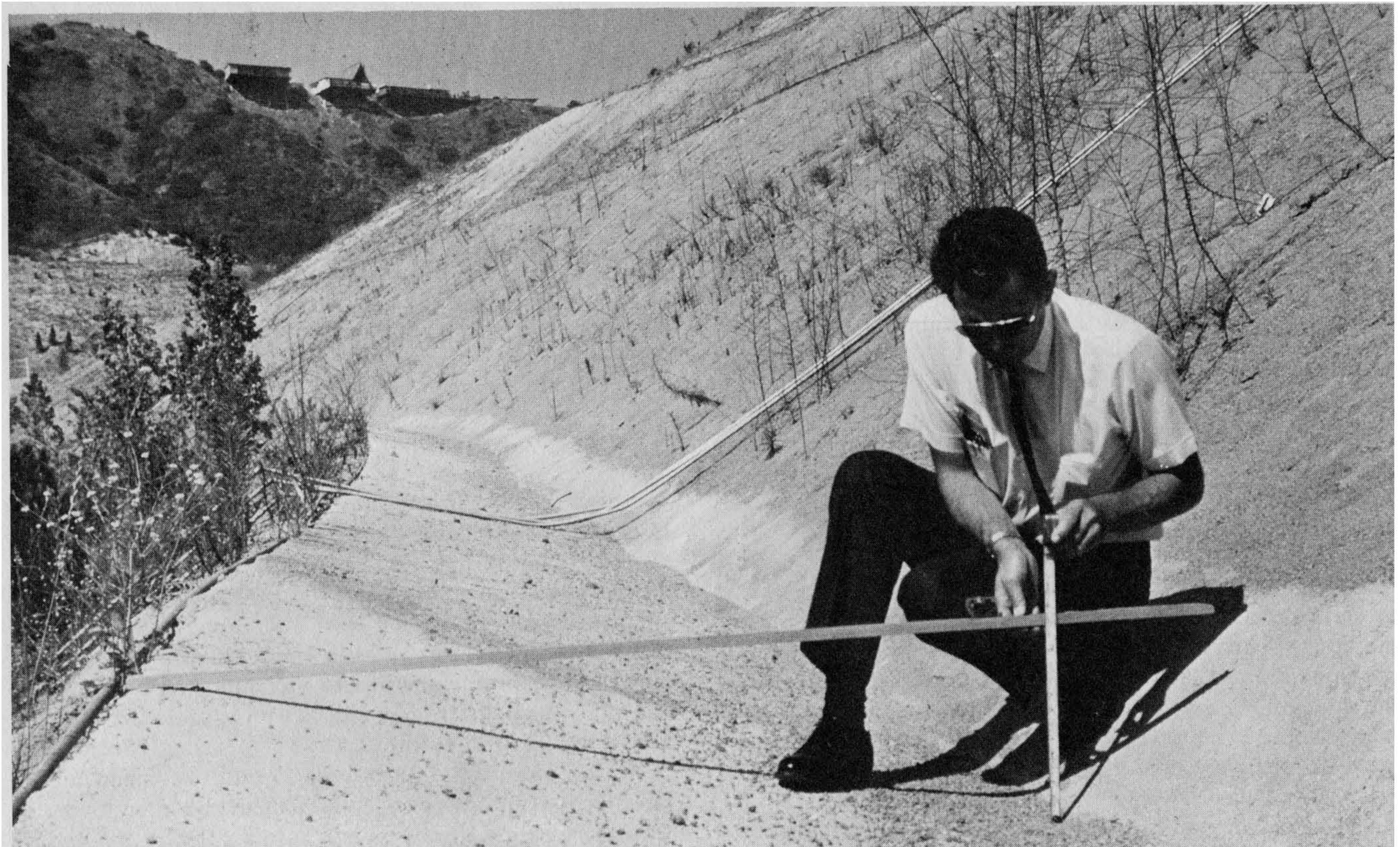
Figure 5-54 Kenyon H. Carr, senior grading inspector, West Los Angeles office, inspects and measures width and depth of terrace and down drains as part of final inspection of slope drainage at the rough grade stage. Photograph by and courtesy of Alex Bruce, senior building inspector, City of Los Angeles, CA.
