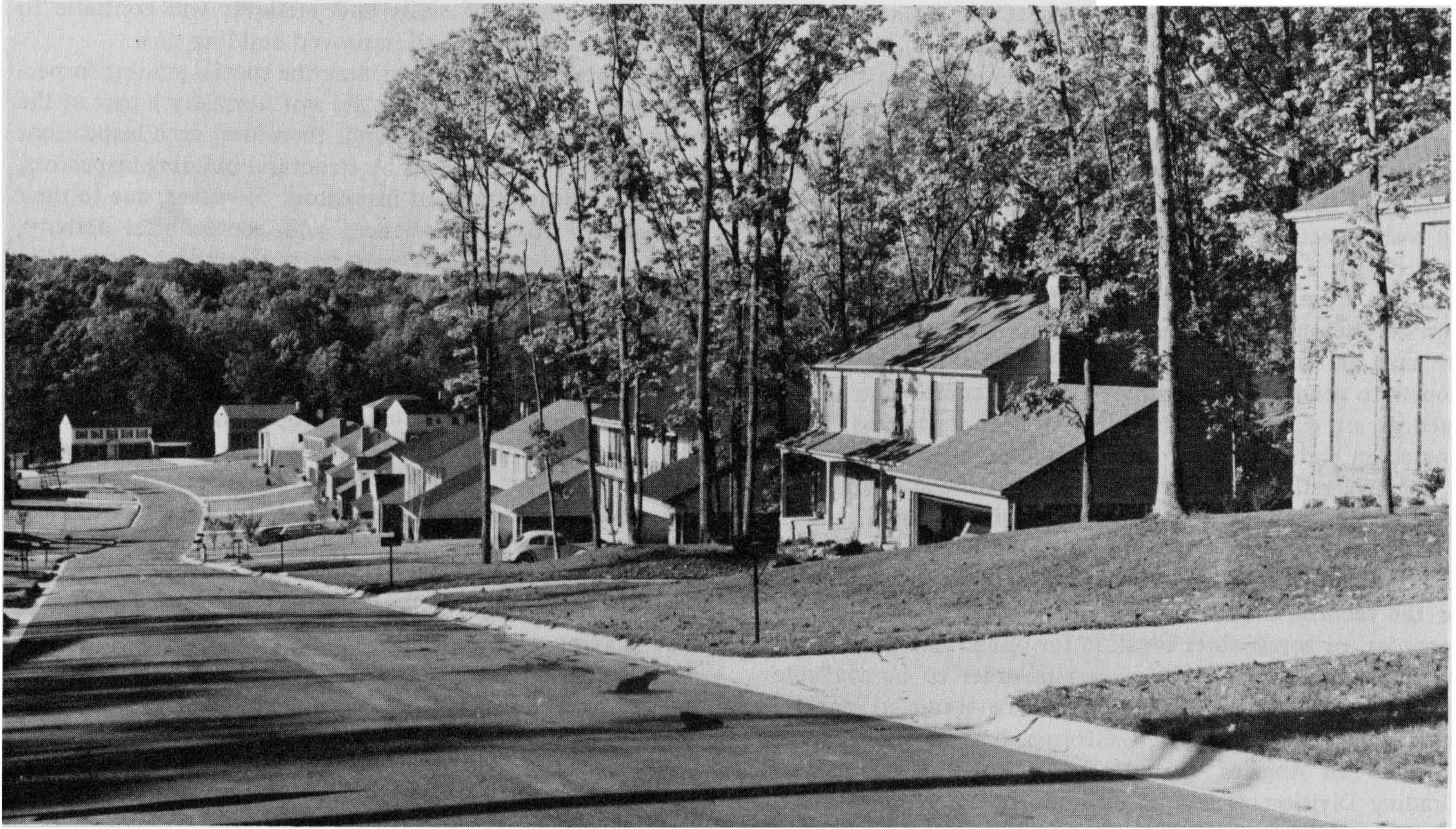
Figure 5-64 A finished subdivision that makes optimum use of existing topography and forest vegetation. Each lot drains readily to the street, and lawns are landscaped to control runoff in an acceptable manner. Photograph by Gordon S. Smith, courtesy of the Soil Conservation Service, United States Dept. of Agriculture.
