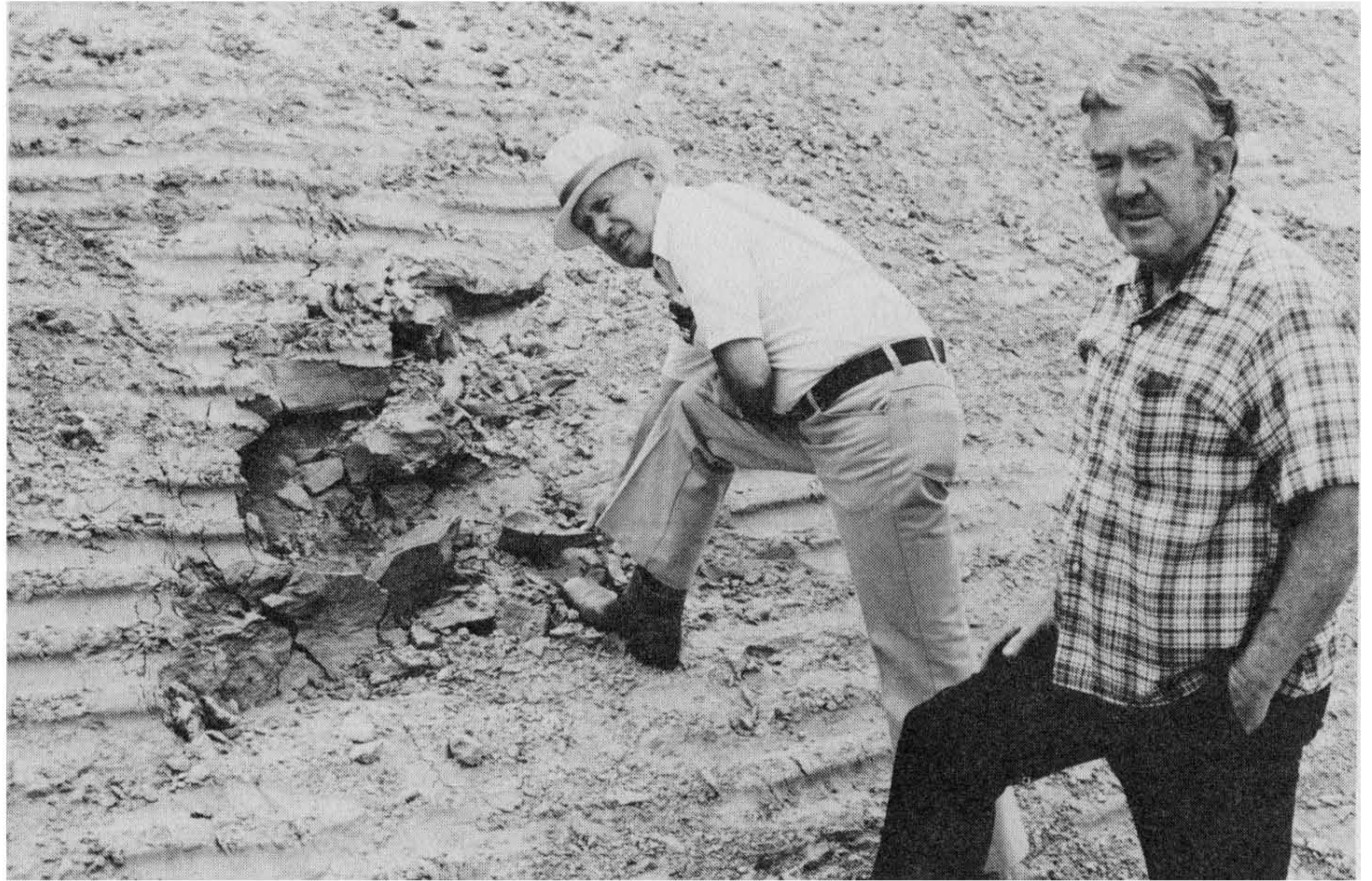
Figure 5-24 A typical toe-of-fill key for the construction of a sidehill fill in siltstone or shale terrain. The toe-of-fill key frequently requires keying and benching through several feet of topsoil, several feet of colluvium, and several feet of bedrock creep in order to key into competent bedrock. Toe-of-fill keys 10-20 ft. deep are common in such areas. Note that the effective bearing point of this toe of fill (45° from the horizontal) moves laterally downslope from the proposed grading plan toe. Source: C. Michael Scullin.
