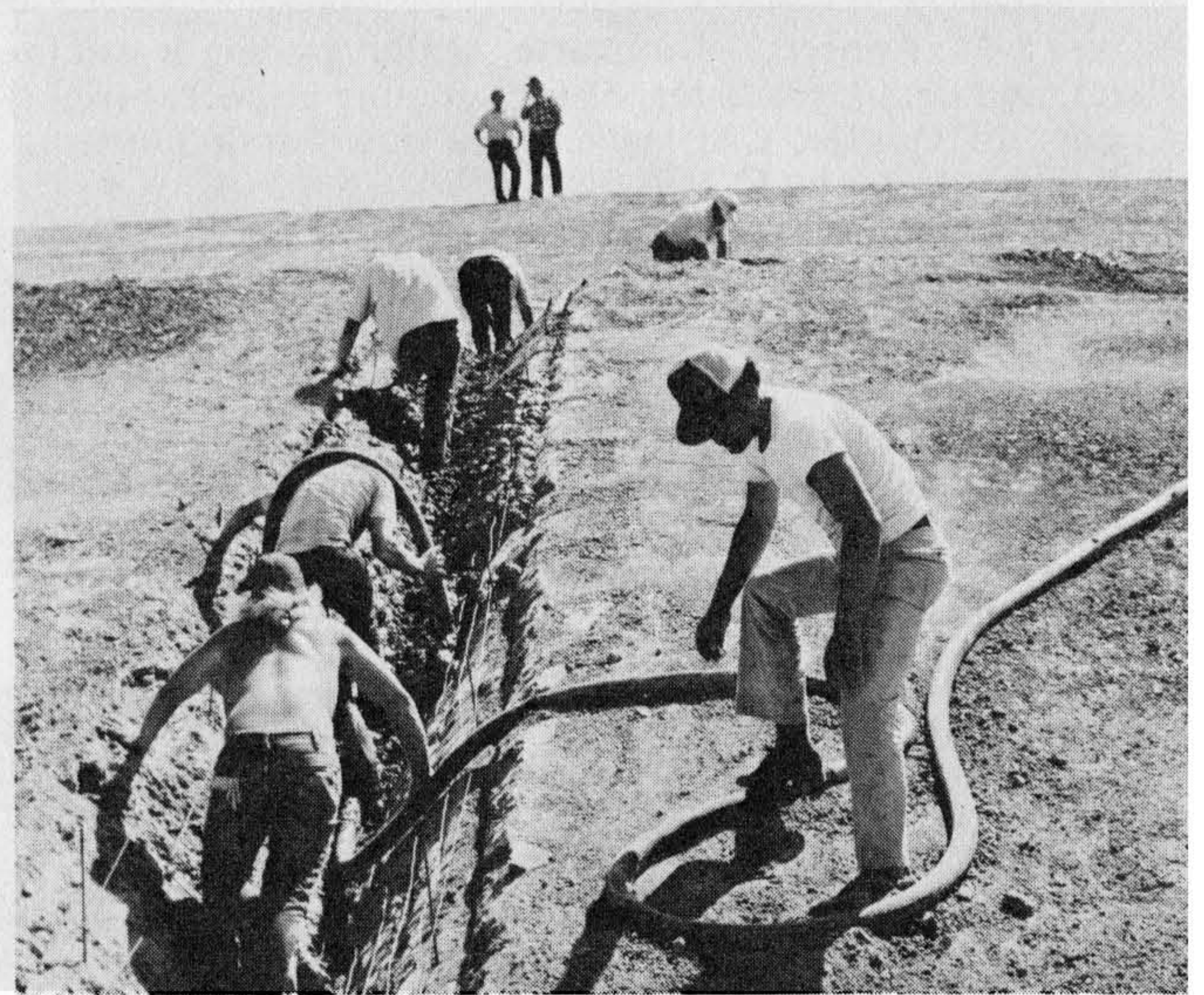
the terrace acts as a cut-off wall for drainage flowing down slope. (c) Guniting the down drain and anchors. Notice that the wire mesh reinforcement is pulled up off the ground surface and is well within the paved section. (d) Guniting the down drain. Photographs by C. Michael Scullin.
