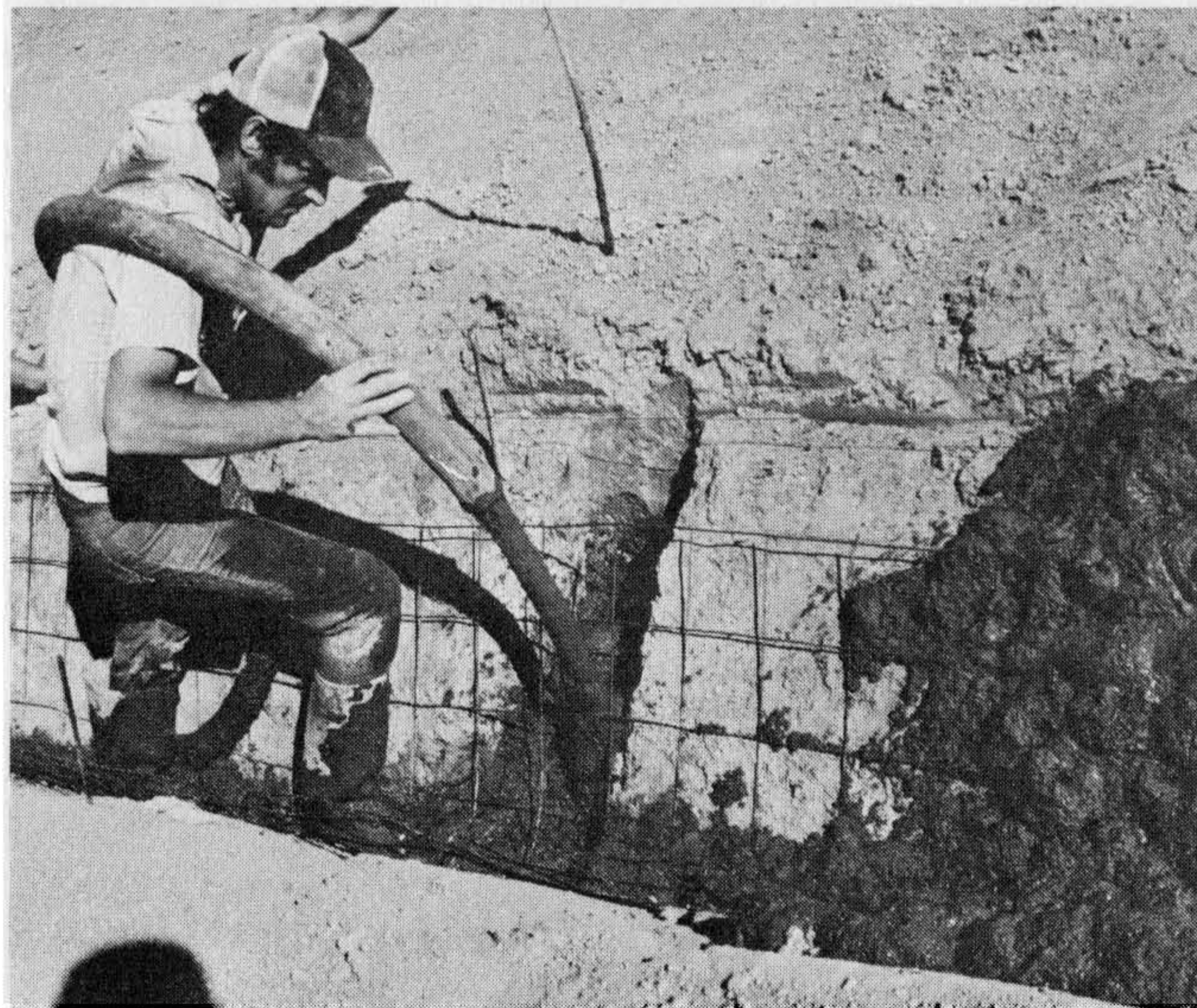
Figure 5-51 (a) Gunite is shot or hosed onto the terrace. The wire mesh should be lifted with a hook rod as gunite is placed to assure that the mesh reinforcement is within the gunite and is not pushed to the bottom by the weight of the gunite. (b) Guniting of this terrace drain is near completion. The surface is finished with a flat trowel and broom. The 4- to 6-inch vertical cut along the backslope (at left) of
