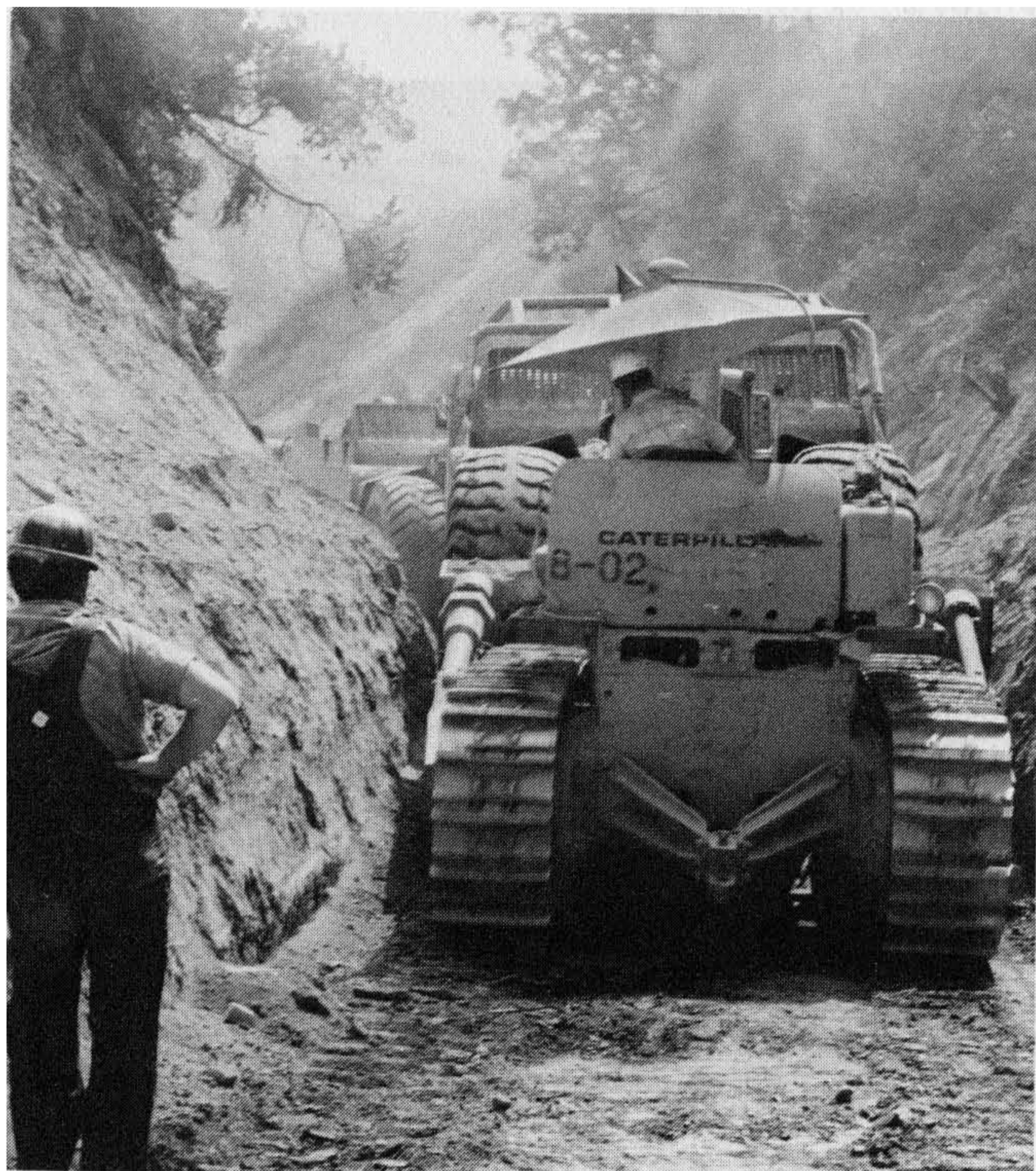
Figure 5-4 Lateral canyon clean-out. The push-cat is pushing the scrapers to assist them in loading. Photograph by and courtesy of Frank E. Denison, geologist.
