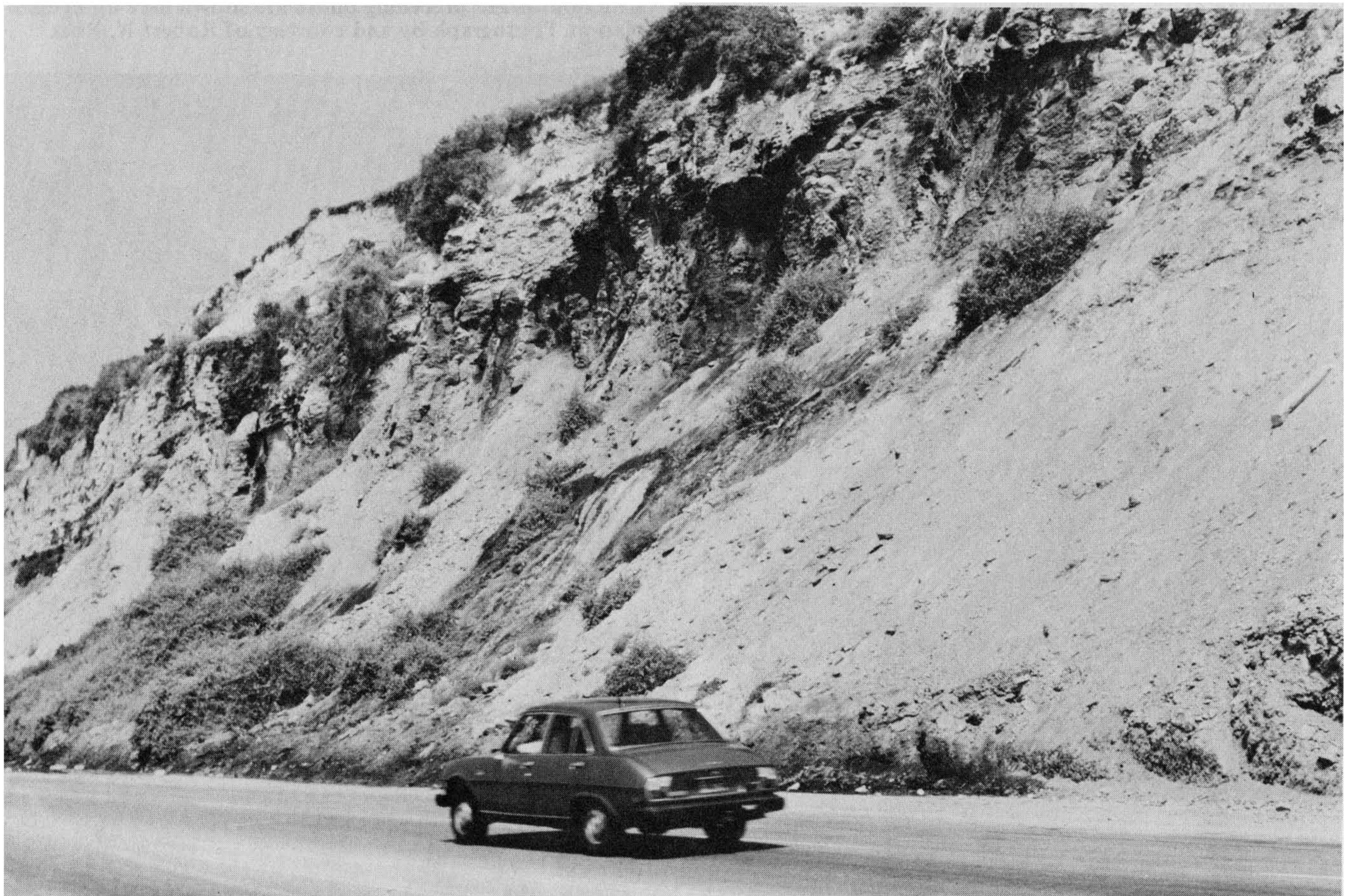
Figure 6-41 Seepage along the coastal bluffs contributes to slope failures. Residential seepage pits located near the top of slopes contribute to water buildup. Photograph by C. Michael Scullin.
