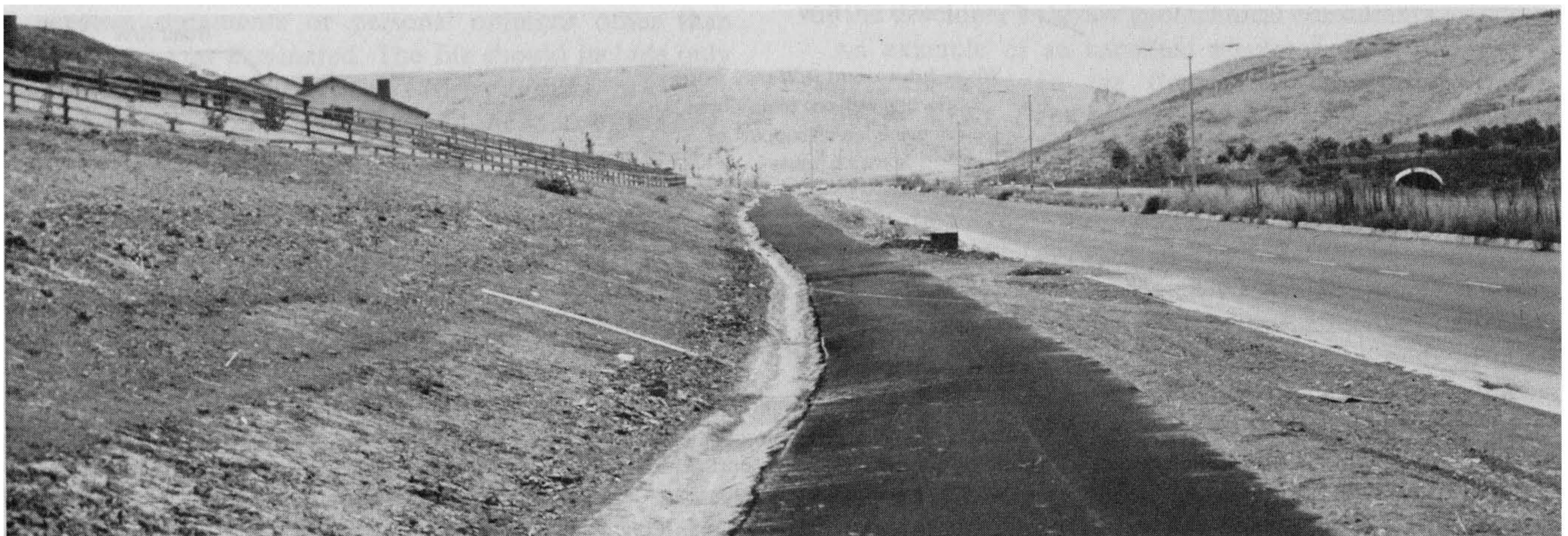
Figure 6-49 This bicycle-skate walk adjacent to a public road has a paved drainage swale at left to protect the paved walkway from erosion. Photograph by C. Michael Scullin.
