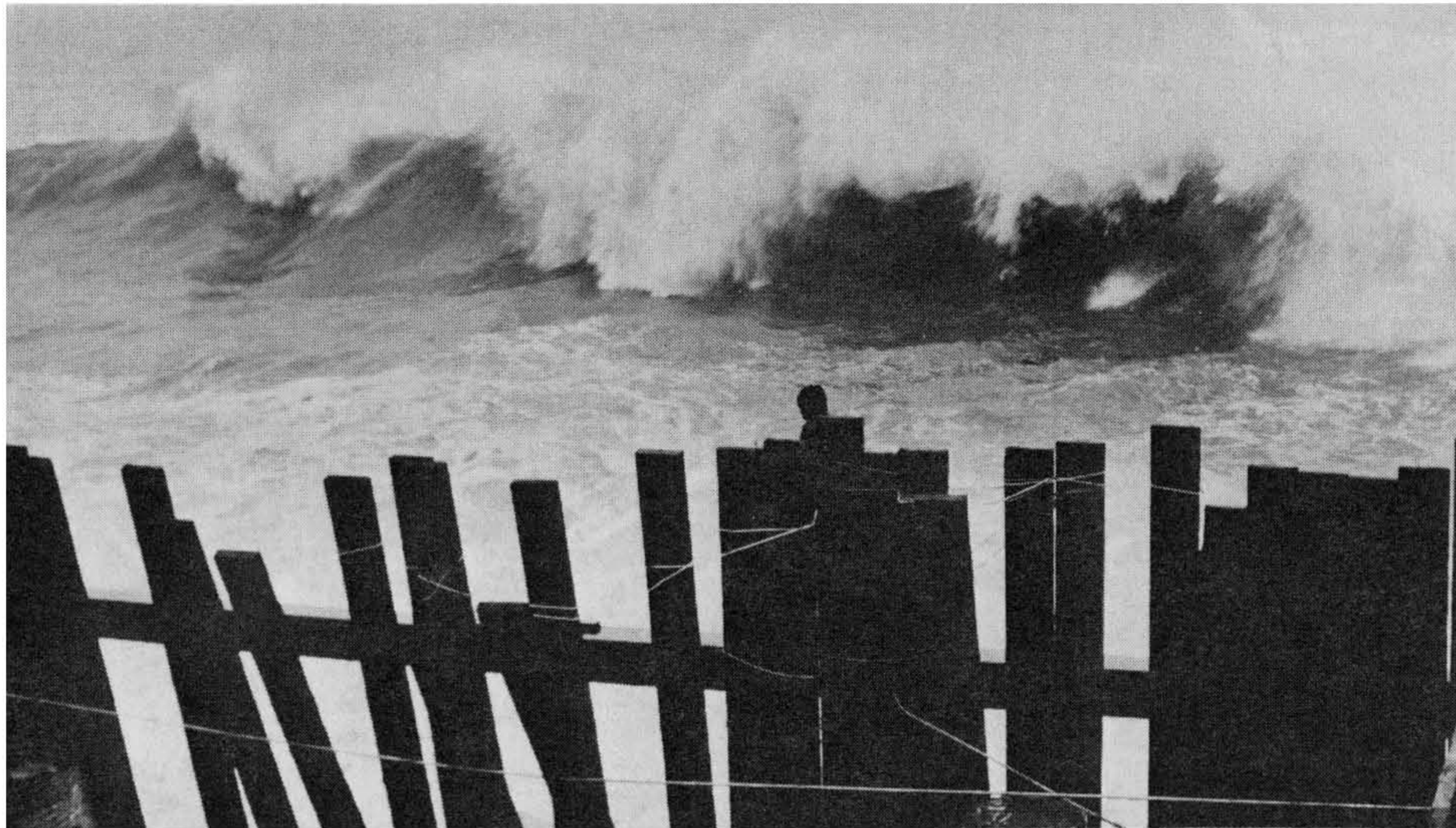
Figure 6-36 Pacific surf is shown pounding and destroying a recently completed wood plank bulkhead which lacked backfill and provided little resistance to the lateral force loads exerted by the ocean. This builder gambled and lost. Photograph by and courtesy of Frank E. Denison, geologist.
