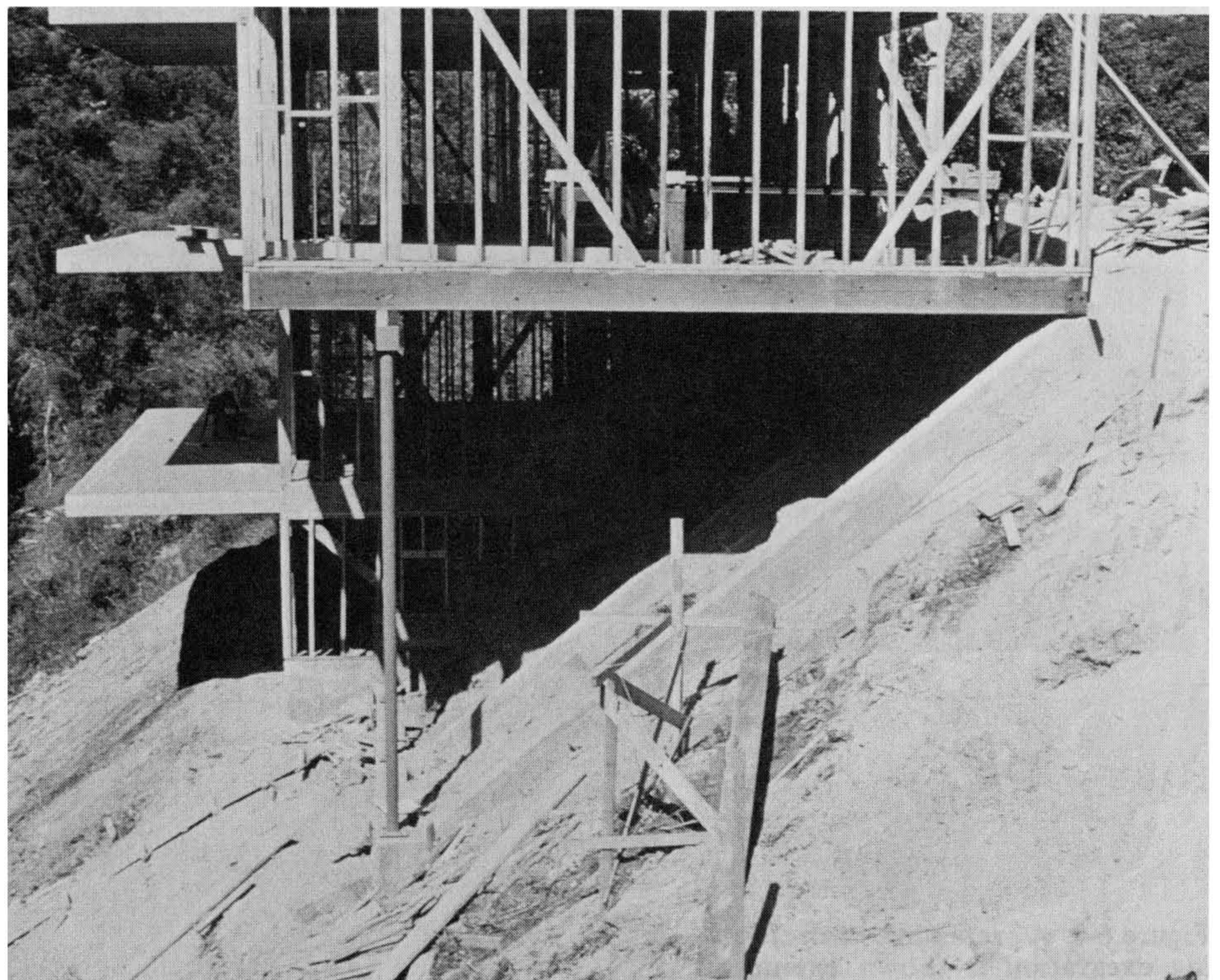
Figure 6-10 Typical cantilevered residential construction founded upon caisson and grade-beam foundations. Such foundation and grade beam designs must provide for the near-surface lateral force loads exerted by down-slope creep. Photograph by and courtesy of Alex Bruce, senior building inspector, City of Los Angeles.
