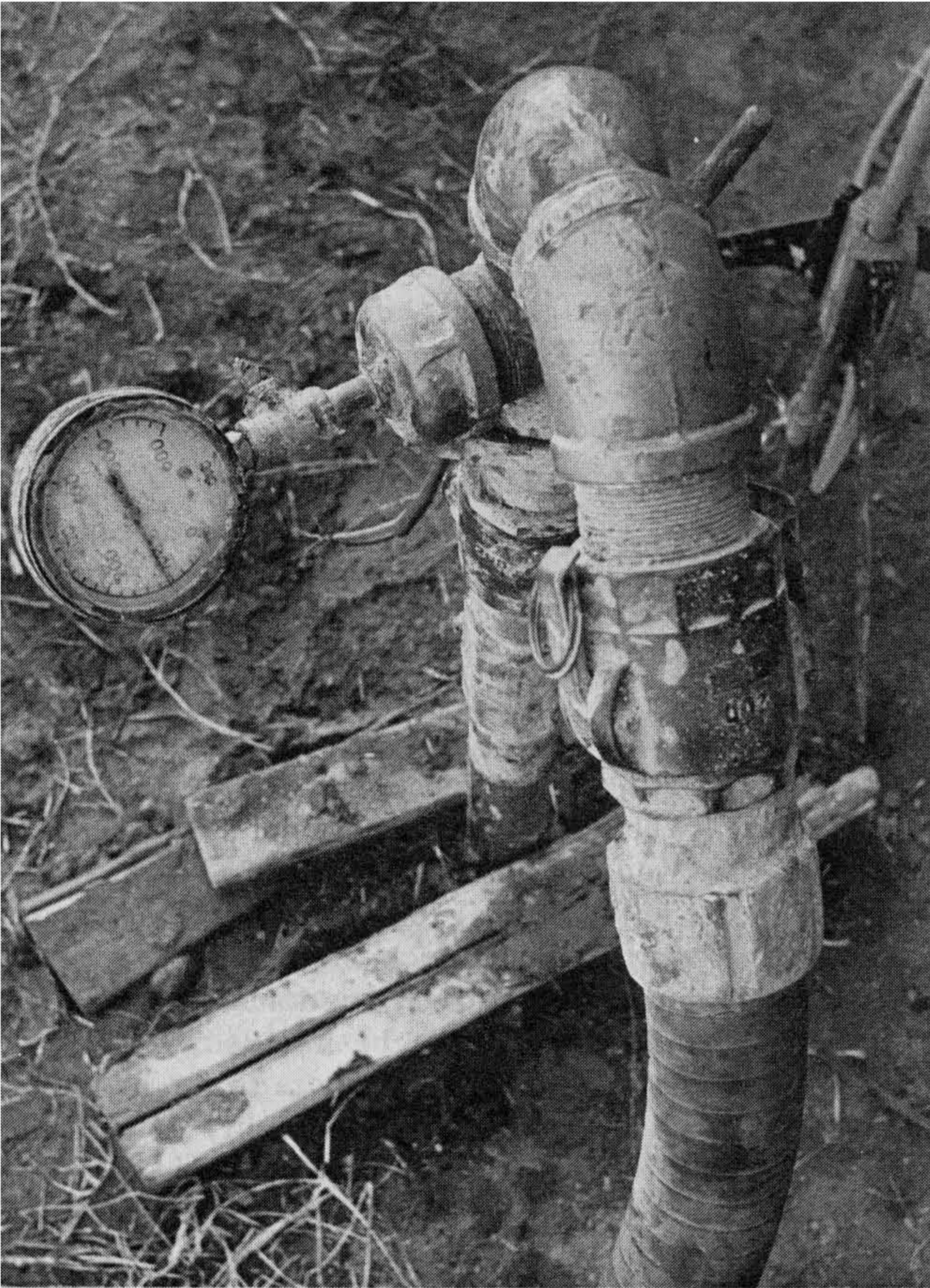
Figure 6-33 (a) A grout injection point with pressure gage is shown. (b) Pumping with a manometer at the front injection point to record ground movement. Photographs by the Los Angeles County Dept. of the County Engineer-Facilities Photographic Unit, courtesy of Jack Eagen, Moore & Taber, Anaheim, CA.
