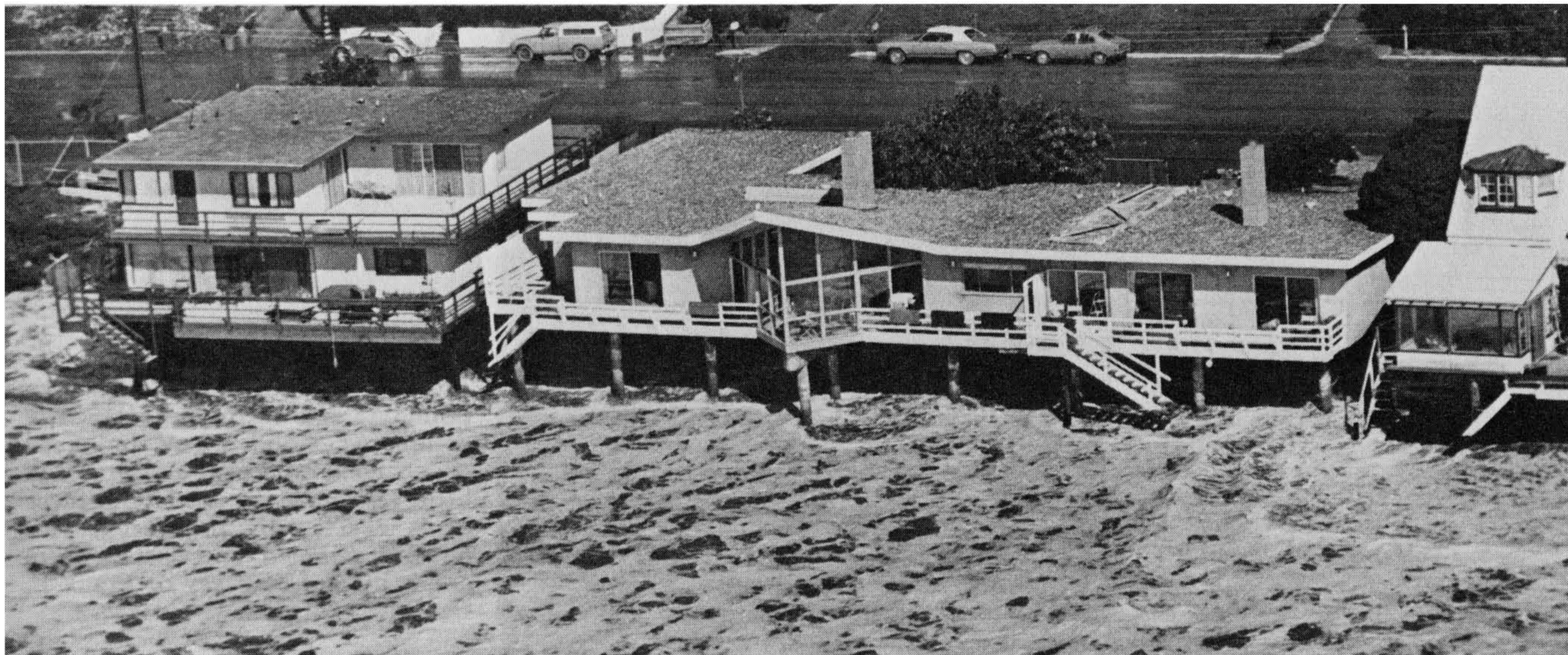
Figure 6-34 Beachfront homes in Southern California with high-tide surf surging beneath. These residences are set on pilings without seawalls or bulkhead protection on the seaward side. Photograph by Mark Malone, courtesy of Kovacs-Byer and Associates, Inc., soil engineers and geologists, Studio City, CA.
