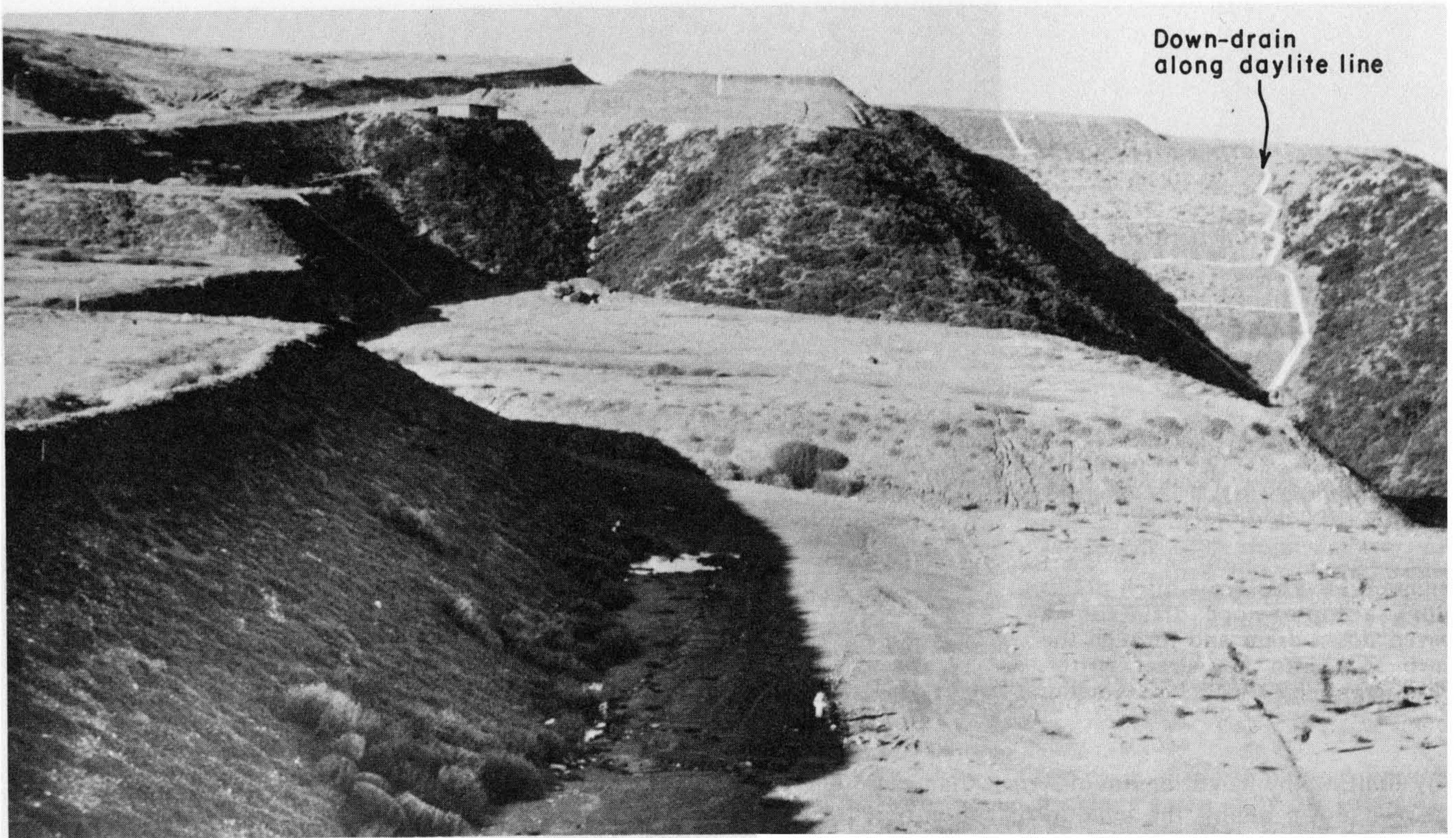
Figure 9-16 The deep V-shaped canyon fill in far right background has down-drains constructed along both daylight lines for better erosion control. Terrace drains are peaked in the center to drain both sides into down-drains. Photograph by and courtesy of Robert W. Ross.
