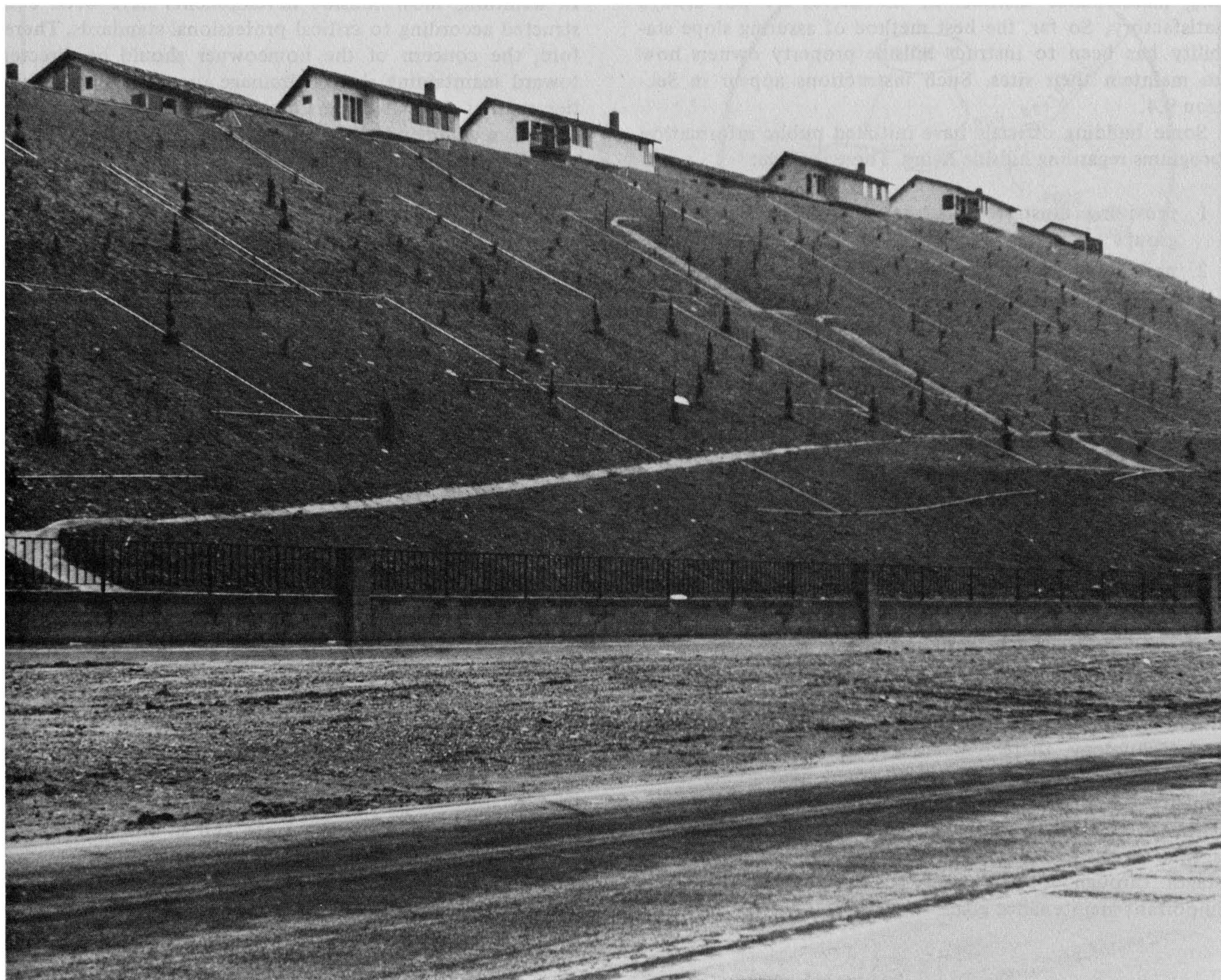
Figure 9-25 A well-compacted fill slope with all drainage devices functioning and minimum water applied. This slope has performed well through three heavy rain seasons. Photograph by C. Michael Scullin.
