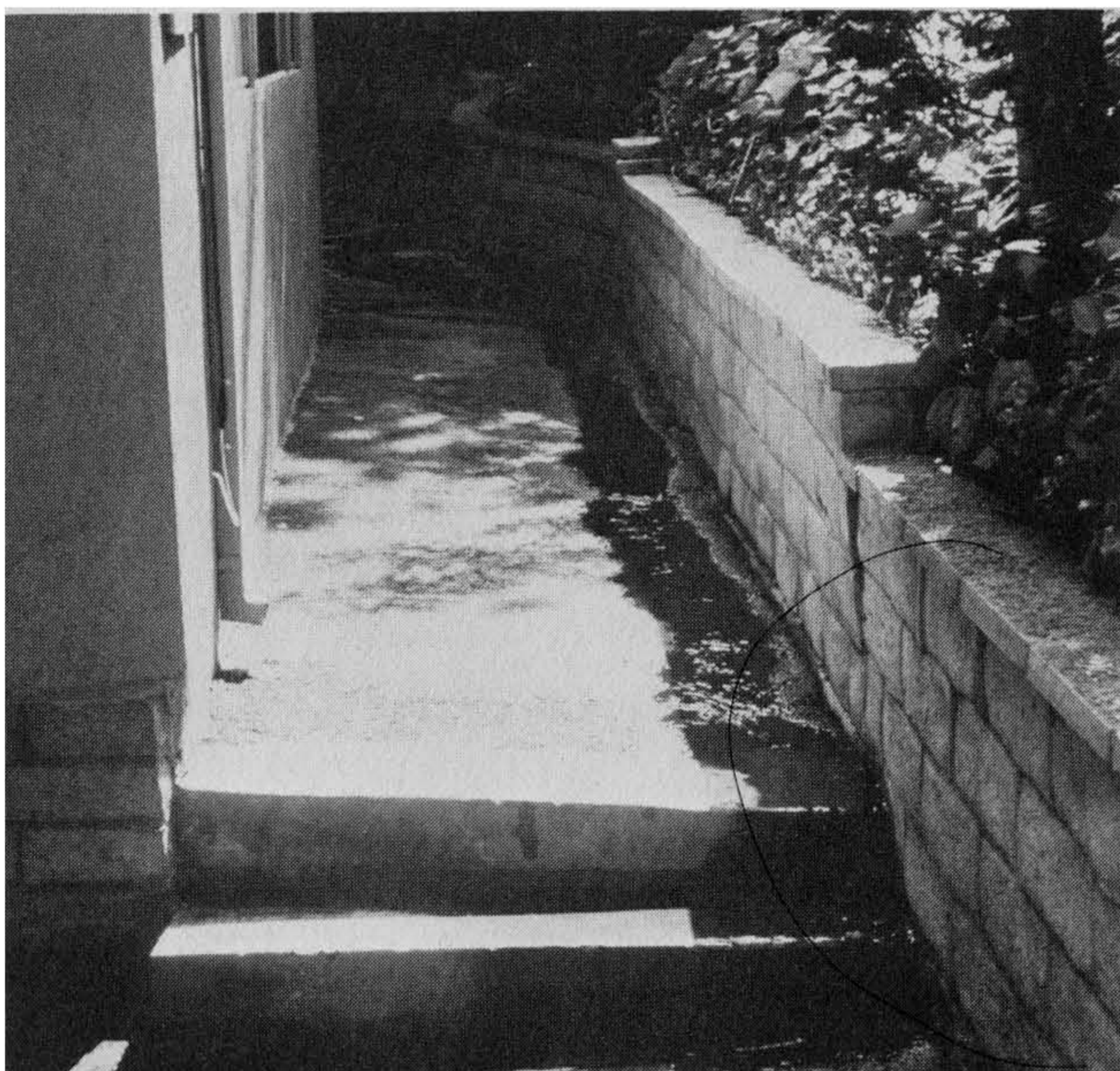
Figure 9-22 This tilted sidewalk drain carries rear yard drainage to the street. Photograph by and courtesy of Alex Bruce, senior building inspector, City of Los Angeles.
