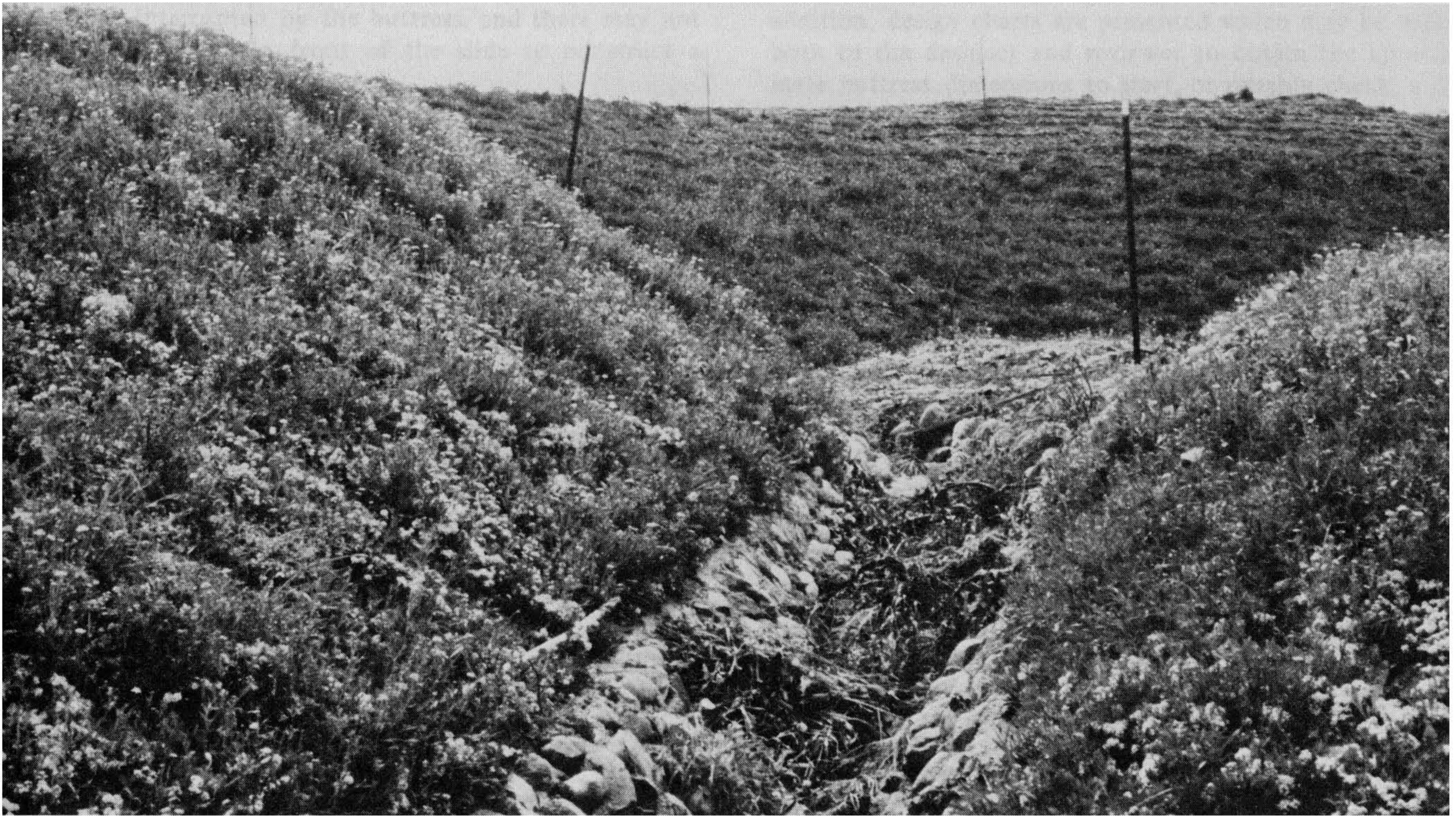
Figure 9-40 The results of twelve months' growth on contoured housing slopes utilizing Rolling Hills Berm No. 43 seedmix. The plant pallette hydroseeding mix has developed fully where the O'Connors legume has formed a
