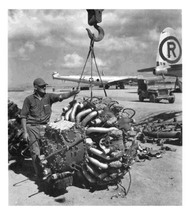
The massive Wright 3350 Cyclone engines that powered the B-29 bomber represented the zenith of 1940s piston engine technology. Each engine weighed 2,800 pounds and employed 18 cylinders, displacing 3,350 cubic inches. The B-29 consumed about four times as much fuel as a B-17 or B-24 bomber.
