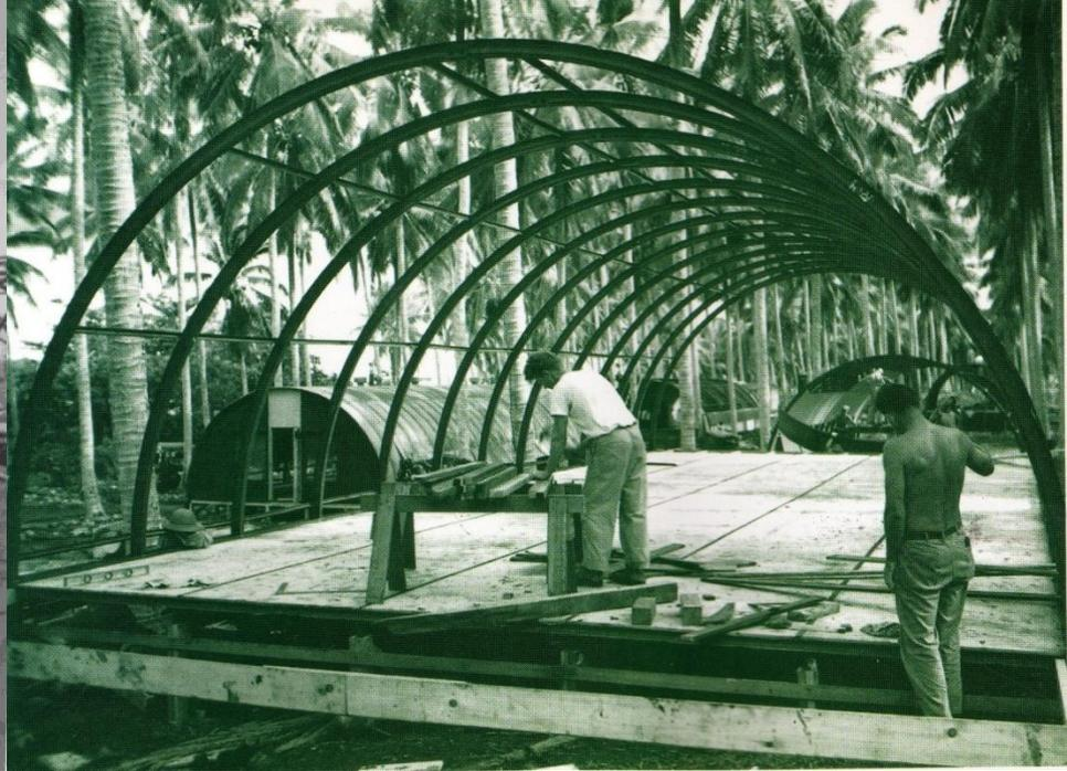
Quonset Huts were known for quick erection of arched **frame ribs** and connecting **purlins**. This shows a hut being assembled on a jig, or erection platform by 33<sup>rd</sup> Naval Construction Battalion in the Russell Islands in Nov. 1943. The exterior sheathing was nailed to the frames and the purlins. After assembly of the frame and exterior sheathing, the unit was moved to its pad (note completed shells in background).
