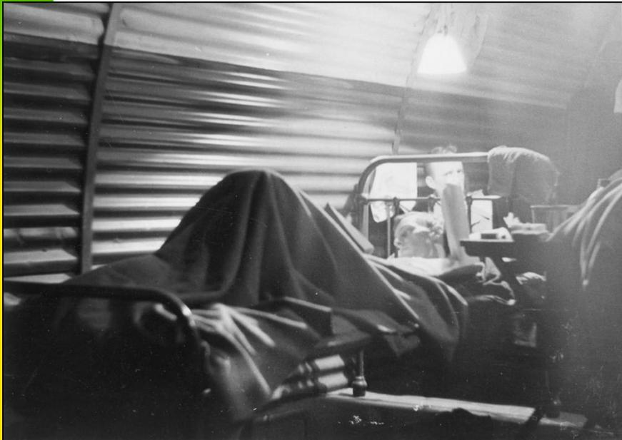
English Nissen Huts were usually constructed without interior insulation or paneling, as shown here (612<sup>th</sup> BS BOQ at Deenethorpe). The lower portion of the sidewalls were painted olive drab, heated by a coal fired pot belly stove, and usually filled with cigarette smoke and perpetual card games between missions.
