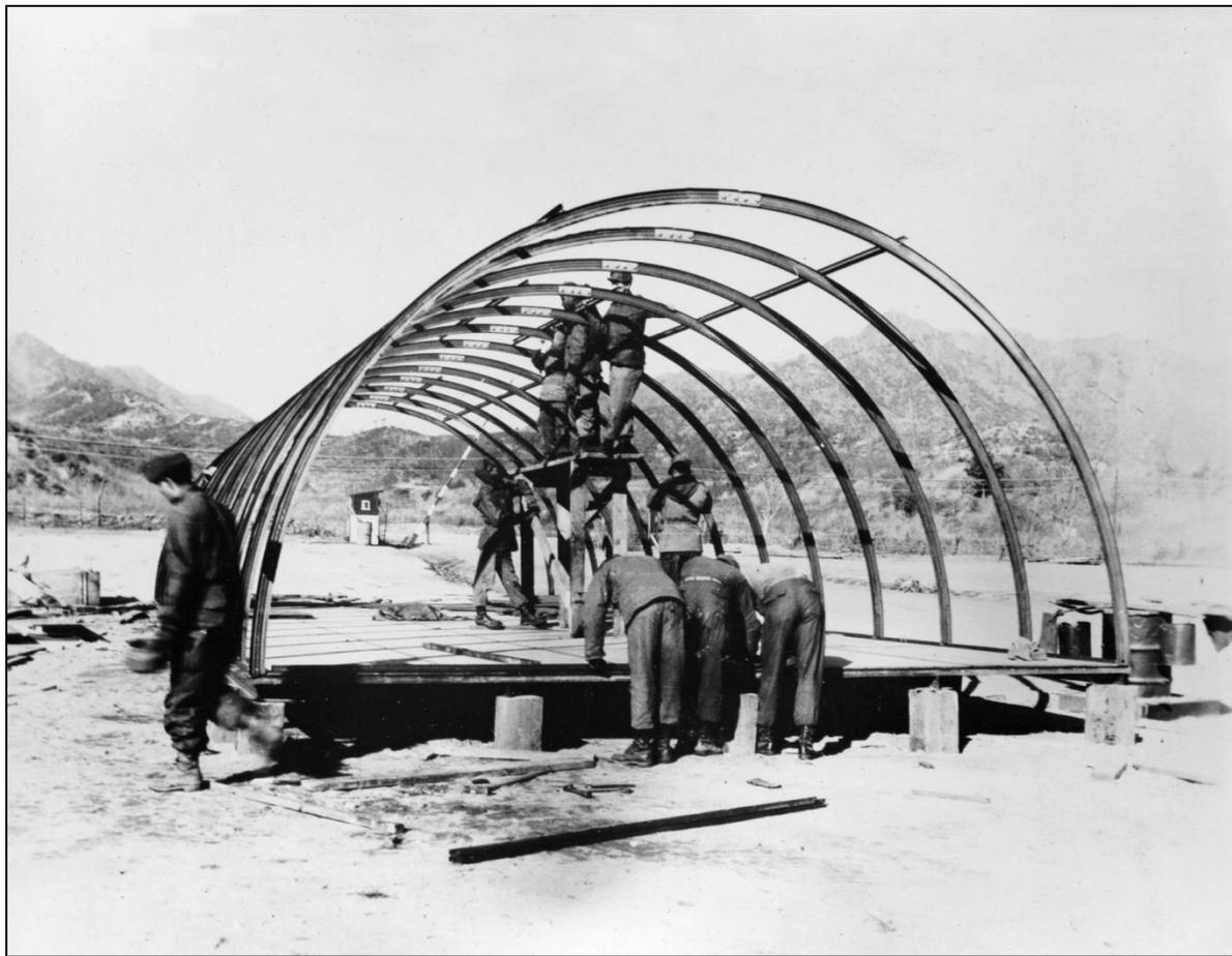
■ The Korean Armistice in June 1953 necessitated the construction of more permanent military bases south of the Demilitarized Zone (DMZ) for American and Korean security forces guarding the border. This shows a standard 20-by-48 hut being erected by Combat Engineers of the US 8<sup>th</sup> Army.
