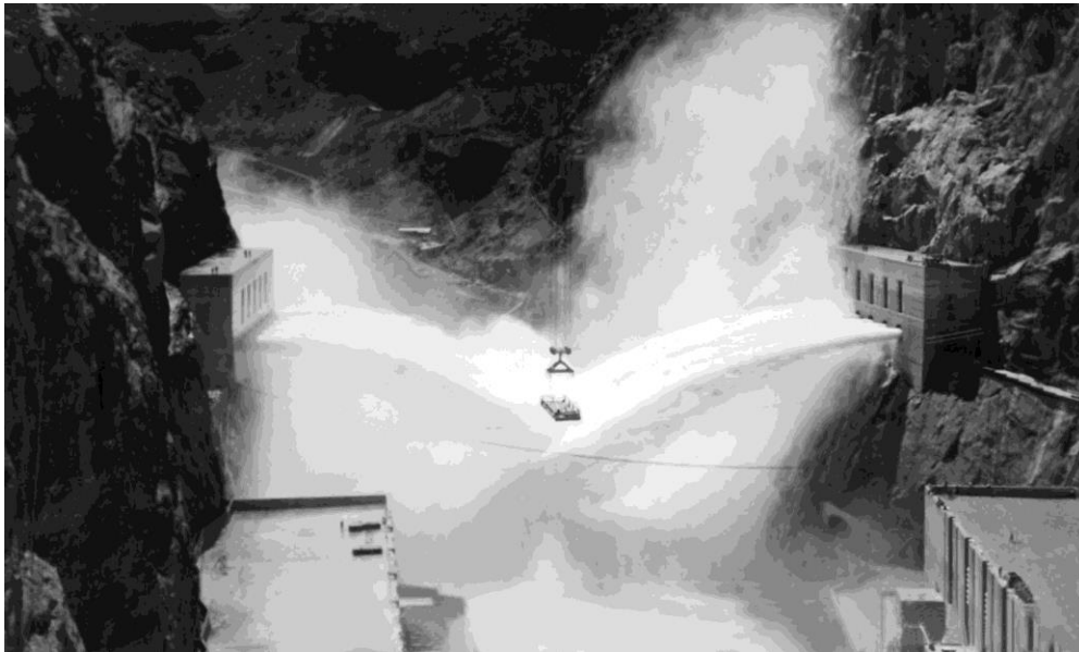
FIG. 17. Water being discharged from the Nevada and Arizona valve houses during the spillway tests in the late summer of 1941, looking downstream (USBR).
