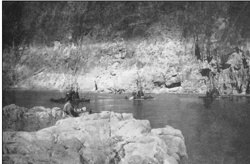
FIG. 11. The Colorado River Board exercised considerable alarm upon their observance of high water marks 80 feet above low water level at the Boulder Canyon dam site (shown above behind rafts supporting three exploratory drilling rigs). This site was near the head of Boulder Canyon. These water marks dropped to about 40 feet above low water by the time the river passed out of the mouth of Boulder Canyon, about five miles downstream.
