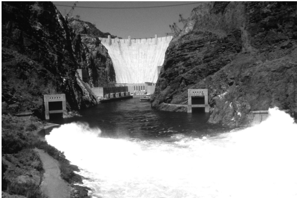
FIG. 8. In July and August 1983 the Nevada and Arizona side channel spillways discharged excess storage for the second time in the dam's history (USBR-LCR).
