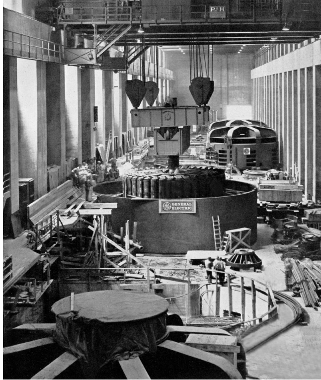
FIG. 3. Gantry crane in the Nevada Powerhouse lowering a 500-ton rotor of Generator N-2, one of the General Electric 82,500 kilovolt-ampere generating turbines, and the first to brought online at Hoover Dam, on October 26, 1936 (USBR).
