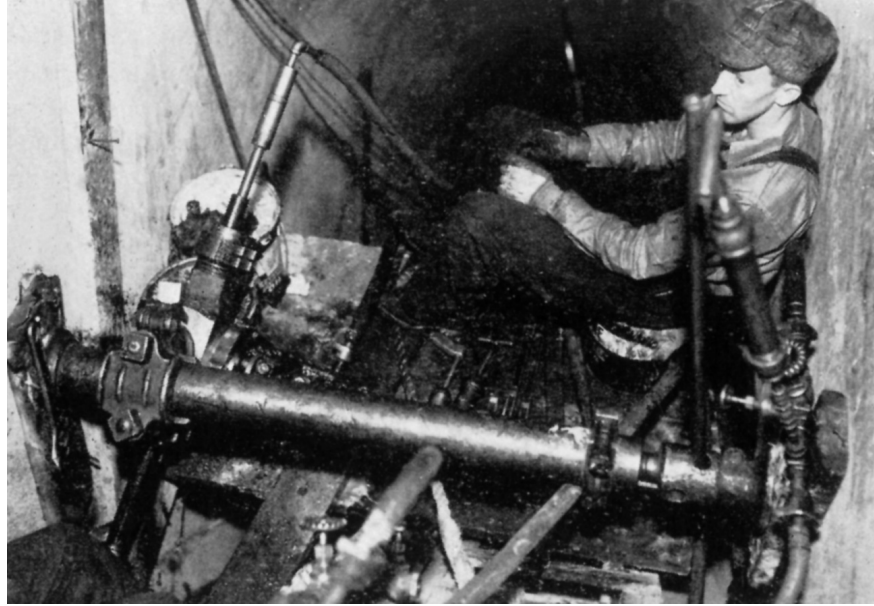
FIG. 15. Cramped working spaces typified the 9- year program of extending the grout curtain, between 1938 and 1947 (USBR).
