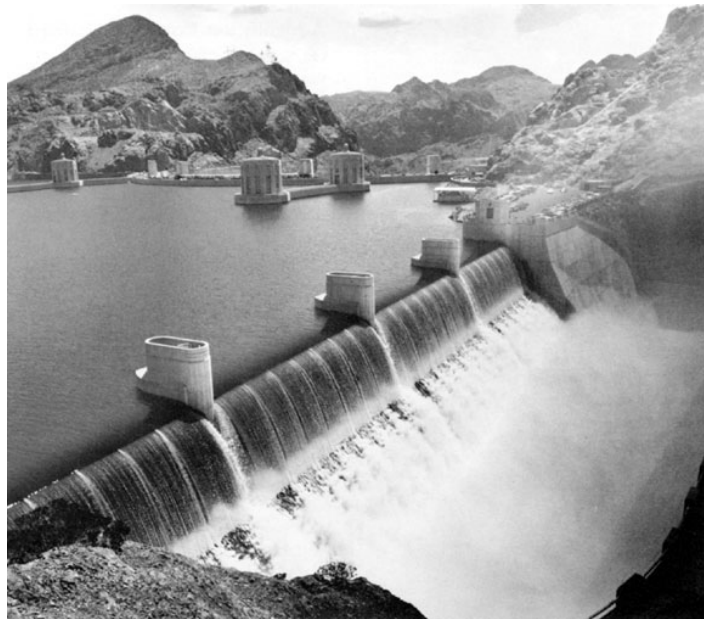
FIG. 5. Water from Lake Mead discharging over the four drum gates of the Nevada spillway during spillway tests in August and October 1941 (USBR).
