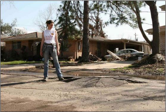
Figure 3.28: Upper photo shows gross near-surface settlement of homes in the Lakeview neighborhood, close to the 17<sup>th</sup> Street Canal breach. Most of the homes were constructed from 1956-75 and are founded on wood piles about 30 feet deep. The lower photo shows protrusion of a brick-lined manhole on Spencer Avenue, suggestive of at least 12 inches of near surface settlement during the same interim (photos by J. D. Rogers).
