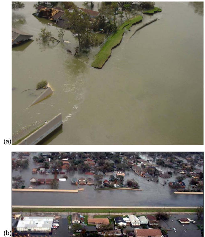
Fig. 10. Upper image provides overview of 17th St. canal breach, looking east. Breach is about 150 m long. Lower image shows oblique view of translated embankment, with intact concrete flood wall at lower left. Land side of levee translated up to 15.85 m, with little vertical differential. One section of concrete I-wall tilted forward (left foreground) while most of wall appears to have been carried entire distance before falling backward, towards canal (upper center). Images from Federal Emergency Management Agency.
