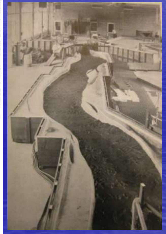
Fig. 6—Much rectification of the high-water channel has been accomplished by setting back the levee line at projecting points, as shown in this stretch between Greenville and Vicksburg.
