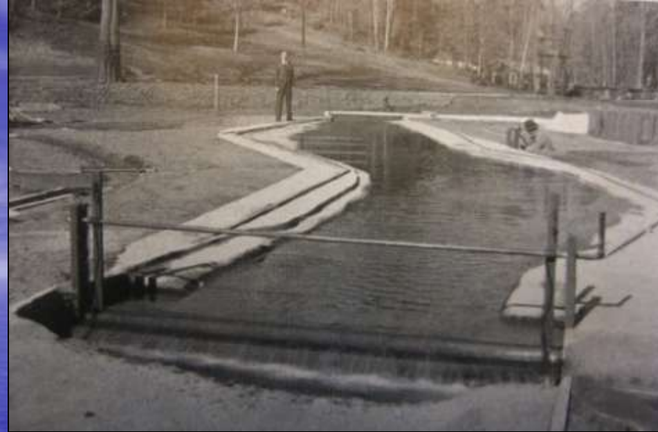
The loess soils in Vicksburg were ideal for carving precise scale hydraulic models, with vertical exaggeration
