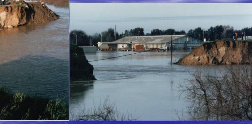
The breach of the Linda Levee along the south side of the Yuba River near its mouth was only 170 feet wide, even after flood waters had poured through the opening for five days.
