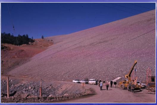
At 770 feet high and 5,600 feet long, Oroville Dam was the <u>highest dam in the world</u> when it was completed on the Feather River in 1967. It was deigned by the CA DWR, with embankment volume of 80 million yds<sup>3</sup>.
