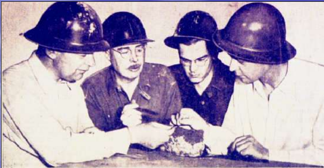
Soil experts find ours good — Dr. M. J. Hvorslev (left), research expert for American Society of Civil Engineers, and Dr. Arthur Casagrande (right), co-founder of new science of soil mechanics, study sample of soft clay taken from Chicago subway, and assure R. S. Knapp and Dr. R. B. Peck that local underground project is "outstanding." (TIMES Photo)
