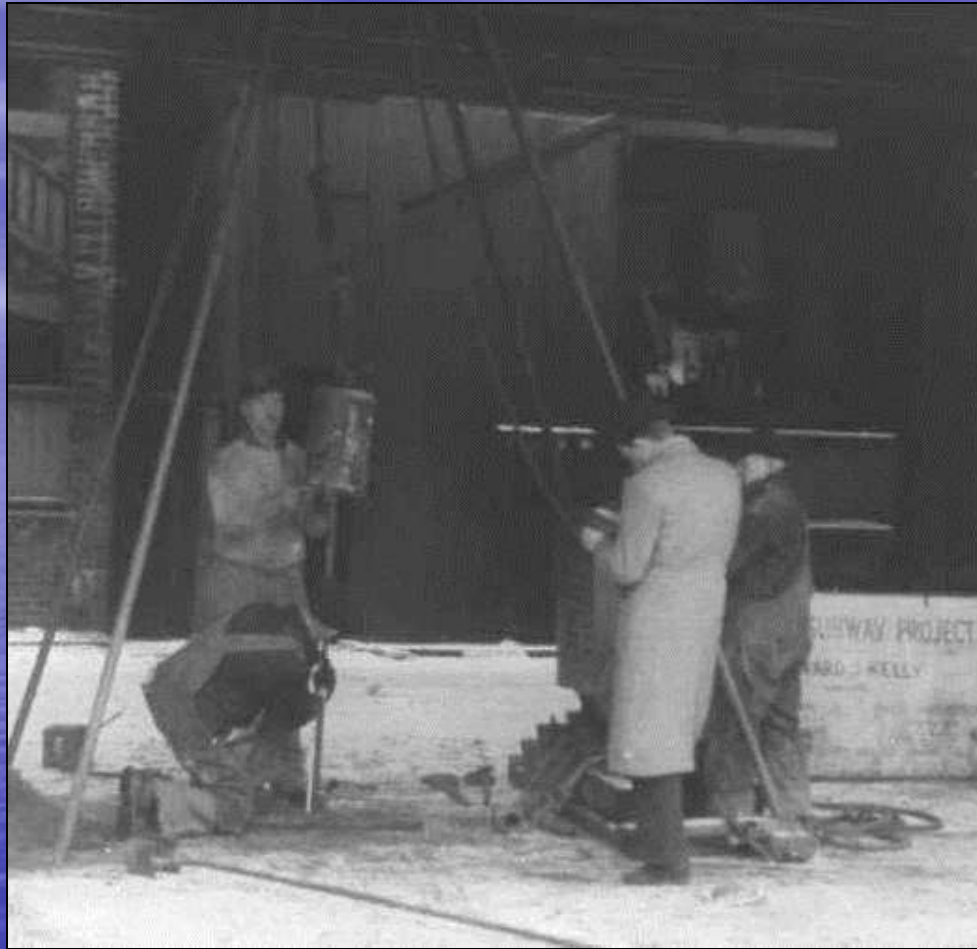
Ralph Peck logging his first soil boring for the Chicago Subway in February 1939 along the State Street Line. Note 140 lb donut weight, employed by the Gow Division of the Raymond Concrete Pile Co.
