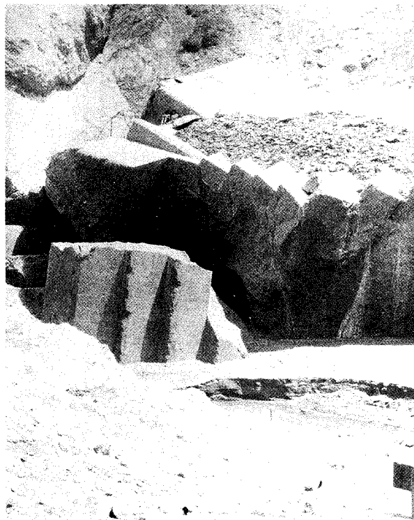
Figure 20. The remains of Blocks 5 and 6, as seen immediately after the failure. The two lowermost steps of Block 1 appear to have been left in tact at the west end. Note the accumulation of schist detritus upon Block 5, about 20 to 30 feet above the creek bed.
