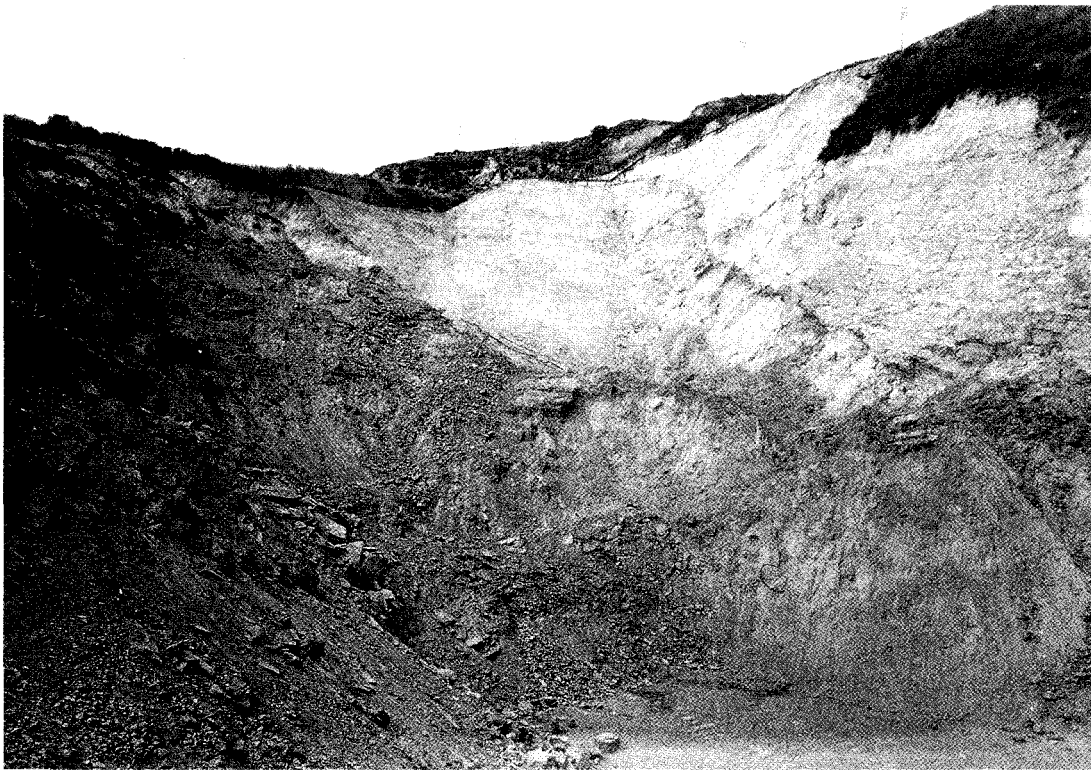
Figure 14. (upper) View looking uphill, into the evacuation scar of the 1928 east abutment slide, as seen from the floor of the canyon, just downstream of the dam's former position. This photo shows the guardrail of San Francisquito Canyon Road, parallel to the slide's west headscarp (thereby fixing its relative vertical position, shown in Figure 15). Photo reproduced by permission of Ventura County Museum of History and Art.
