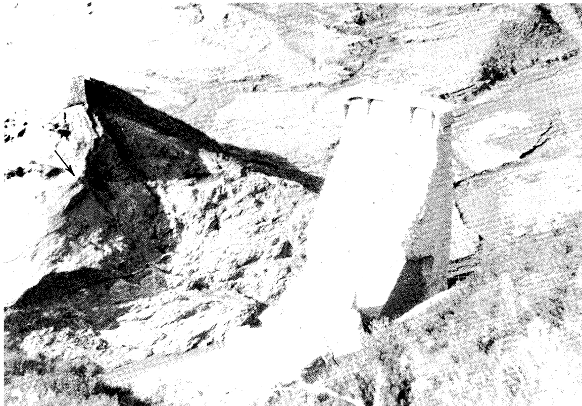
Figure 24. (upper) View looking down on the dam site from the upper surge chamber road (Figure 14 lower) the morning after the failure. Note how the original construction road, leading up to the wing dike, is not damaged above elevation 1785 (arrow). This suggests that, at a minimum, the upper portion of the west abutment did not fail until the reservoir had drained at least 30 to 50 feet (photo courtesy of Ventura County Museum of History and Art).
