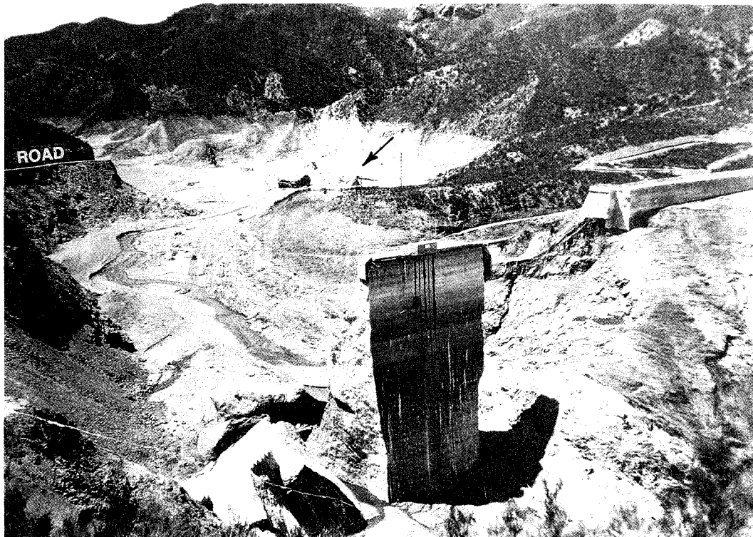
Figure 26. Overview of the flood's aftermath, immediately downstream of the dam. The flood wave scoured the canyon's slopes to a maximum depth of 120 feet above the stream level. The Edison power line crossed the channel, but was situated above the maximum scour line (arrow). San Francisquito Canyon road began climbing east wall of the canyon, at upper left. Photo courtesy of Ventura County Museum of History and Art.
