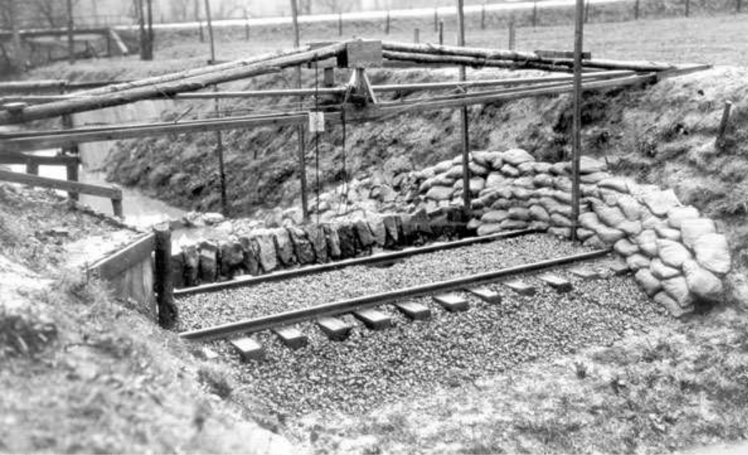
Full-size railroad embankment
