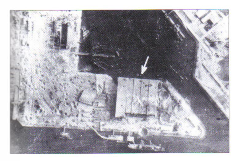
This aerial image shows craters caused by Allied air attacks before emplacement of fangrost covers to absorb bomb detonations.
