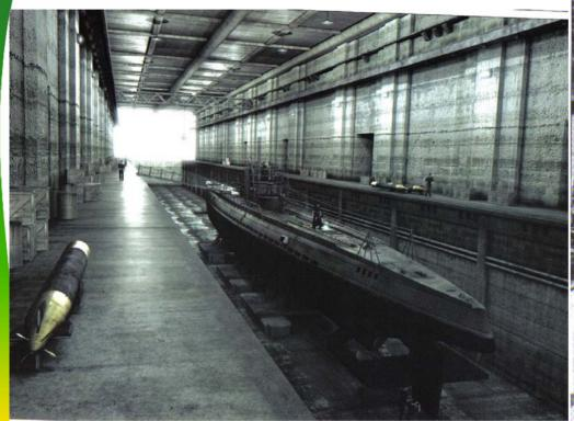
Each pen was designed as a freestanding drydock so essential maintenance and battle damage repairs could be carried out between combat deployments
