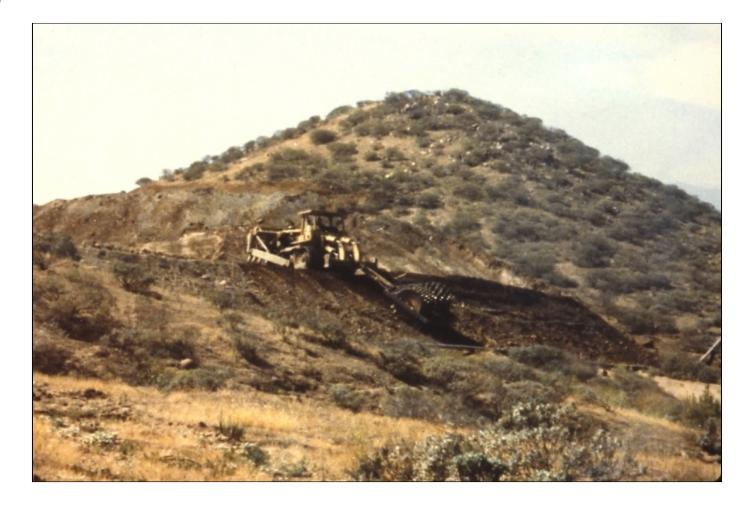
The contact pressure is the roller weight on the teeth multiplied by the cosine of the slope inclination. This results on about an 11% reduction on a 2:1 slope.
