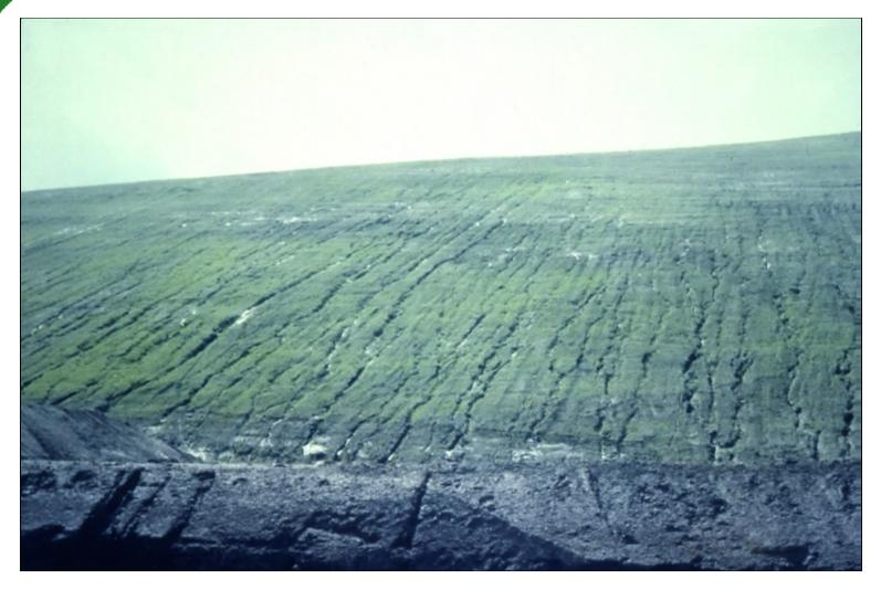
In the 1988 UBC the decision was made to waive the requirement for terrace drains if fill slopes were inclined at 3:1 or flatter. This view shows rill erosion developed on such a slope, despite a healthy grass cover.
