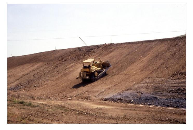
Track walking a fill slope will not compact it appreciably because the track contact pressures are usually between 5 and 10 psi; well below those imparted by a mechanical compactor (>135 psi for pad rollers)
