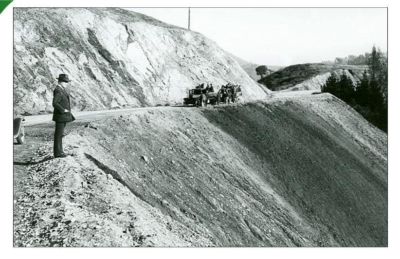
Early fill slopes were typically inclined at about 1.5:1 (33.6 degrees). This shows a sidehill fill slope supporting a newly constructed road along the crest of the hills above Berkeley, CA in late 1934.
