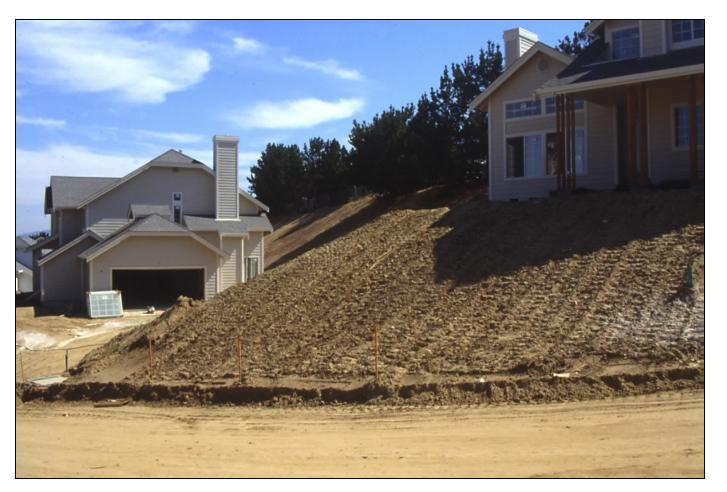
A "dressed slope" is usually walked by a tracked dozer, leaving the track marks. This serrated surface provides superior catchment for hyrdroseeding of most grasses
