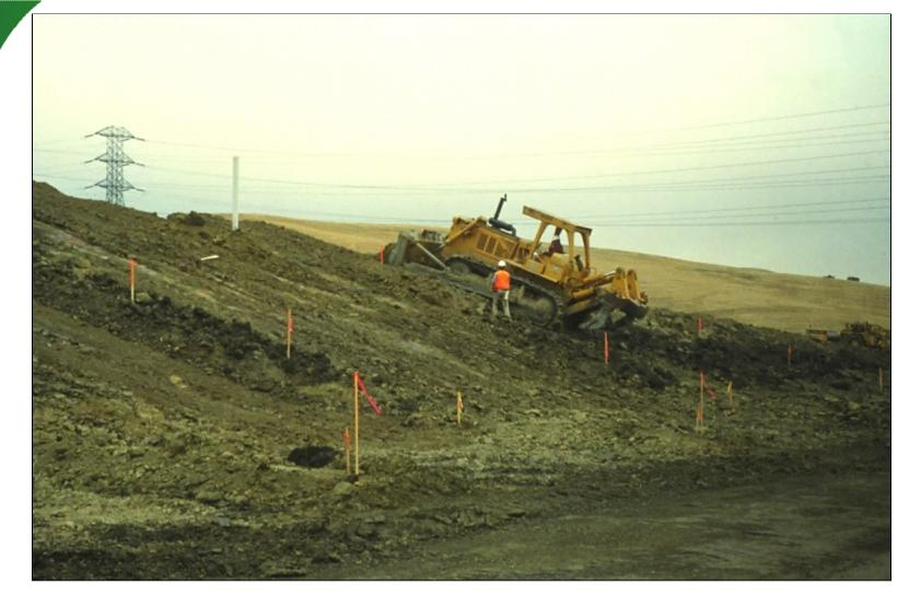
Dressing a fill slope is the process by which the slope is trimmed to its final inclination, as shown here. Note construction staking.
