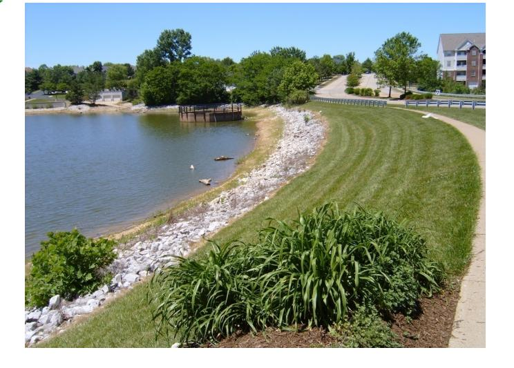
The embankment retaining Lake Chesterfield near St. Louis is typical of many across the humid Midwest, which employ mowed grass and shrubbery for erosion protection.
